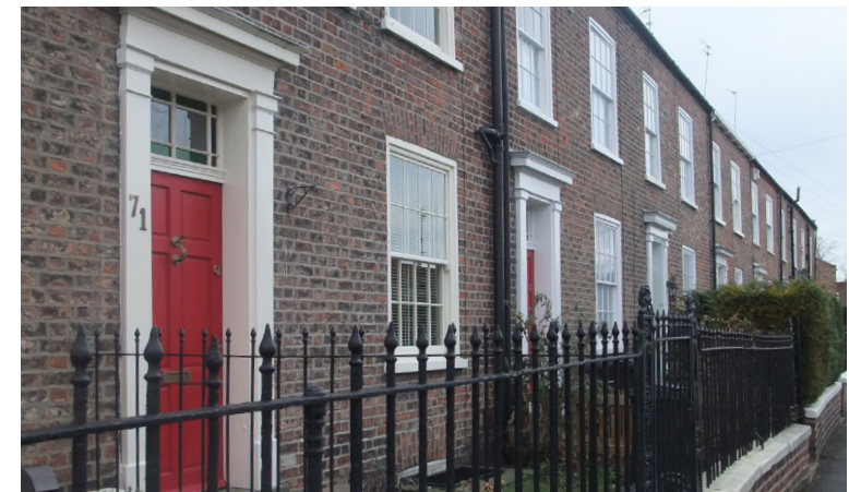
The houses on Union Terrace have small front and rear gardens with the pavement boundary defined by iron railings on low brick walls
