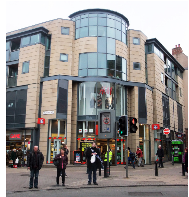
The corner of Spurriergate and High Ousegate is overly complex
