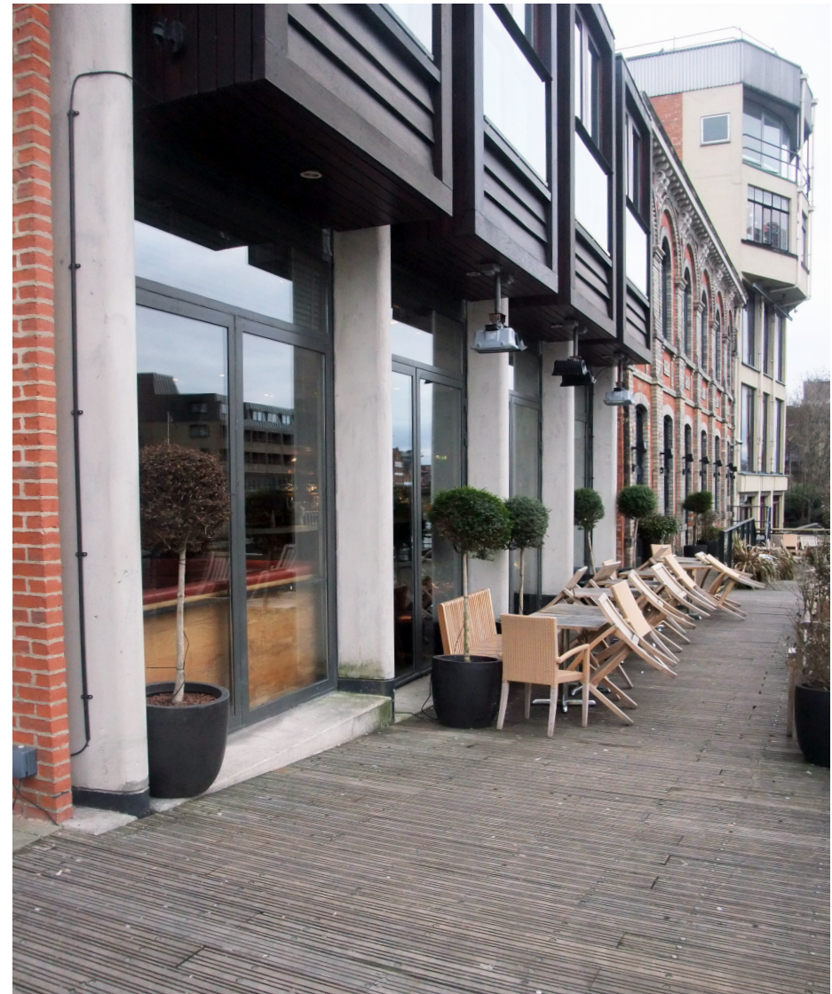
Access to the river is provided by a cantilevered deck, suitable for al fresco dining
