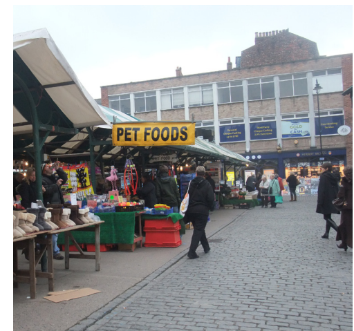
Some of the buildings facing Newgate Market are of poor quality and detract from the space
