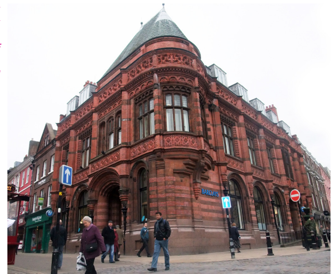
Nos. 1, 2 and 3 Parliament Street is a red brick Gothic building built about 1901 as a bank (current Barclays Bank). The style is an interesting departure from the favoured classical style of many banks, using terracotta and ceramic panels instead of stone. The building is Grade II listed
