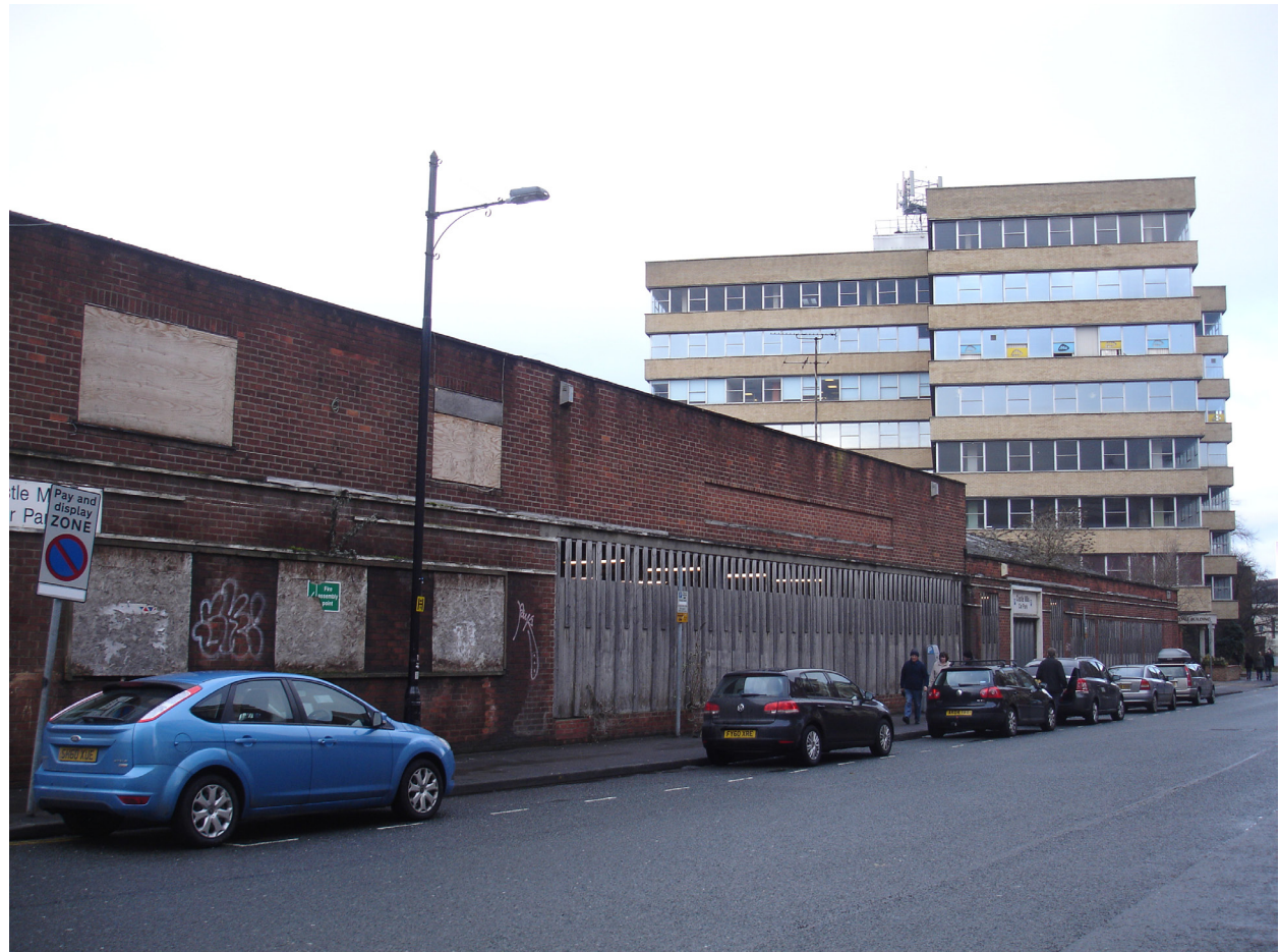
View of Ryedale House from Piccadilly, with run-down single storey warehouses in the foreground
