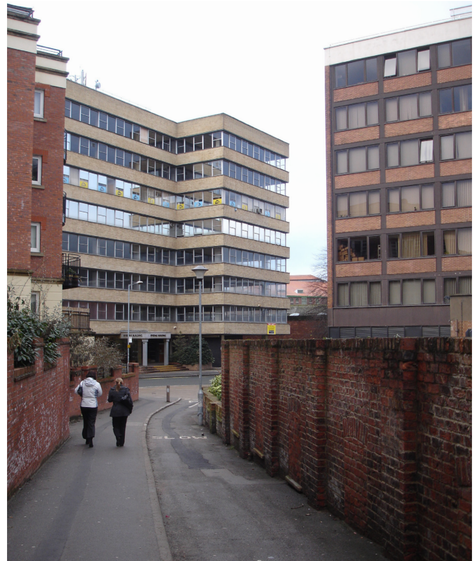
Ryedale House blocks potential views to the Castle from Dixon Lane and Piccadilly
