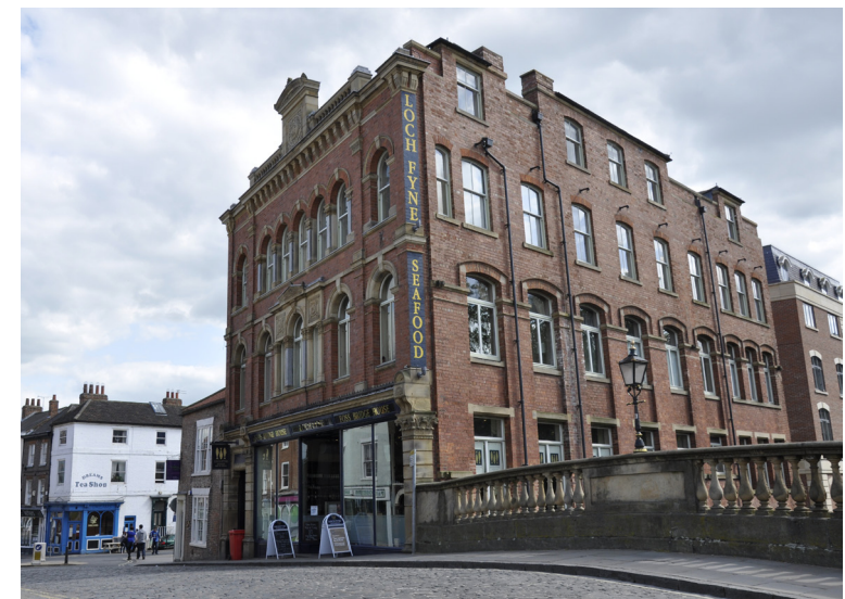
The warehouse of linen and woollen traders W.G. Whitehead and Co
