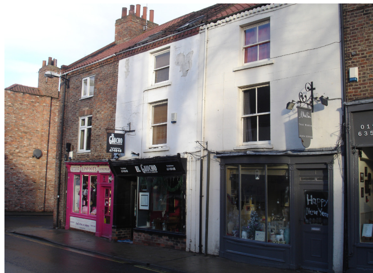
A group of houses converted to shops on Walmgate
