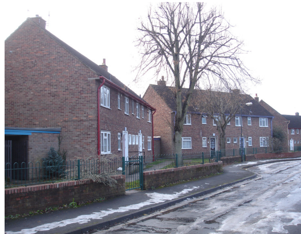
Blocks arranged in a 'zig-zag' along the street on Long Close Lane
