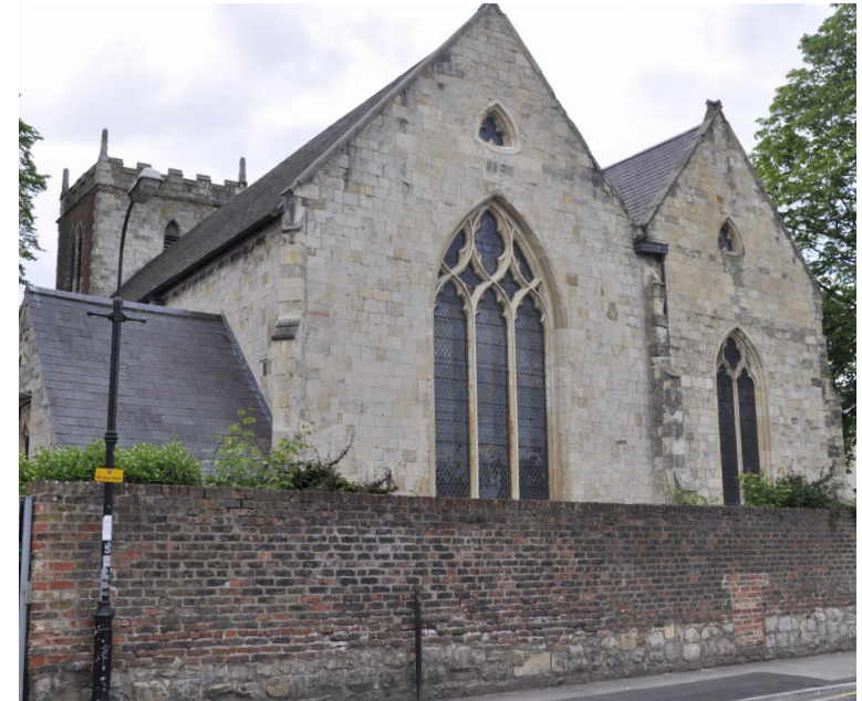
Grade I listed medieval church of St Margaret's on Navigation Road
