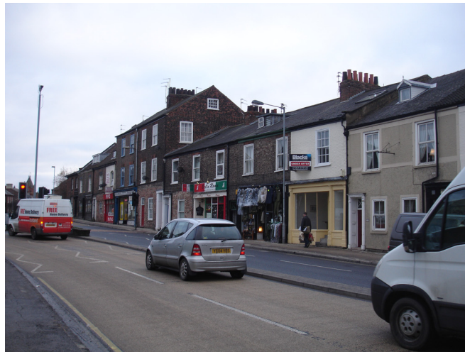
Some houses on Fishergate have been poorly converted into shops and much altered
