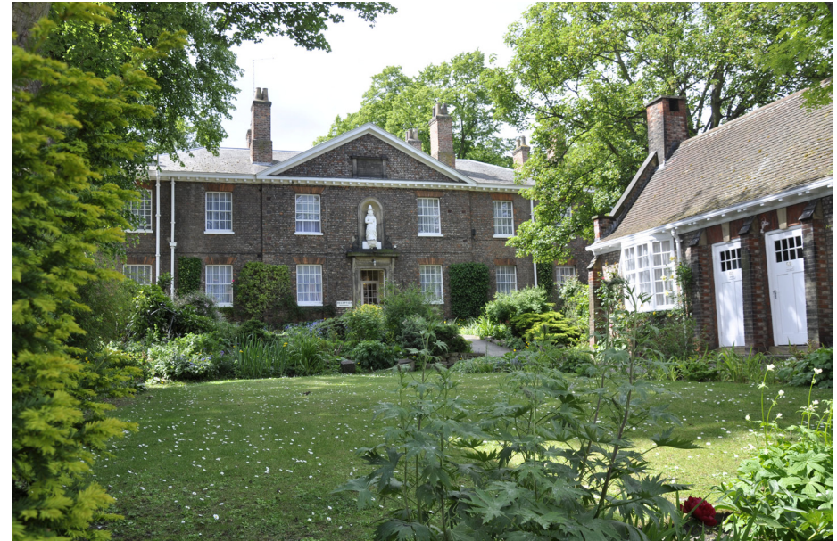
Lady Anne Middleton's Hospital is set back behind an attractive garden. Built 1827-9 by Peter Atkinson junior. Grade II* listed and now a hotel
