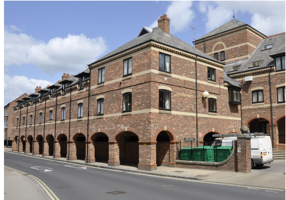
Parking is accommodated on ground floor in modern apartment blocks on Skeldergate
