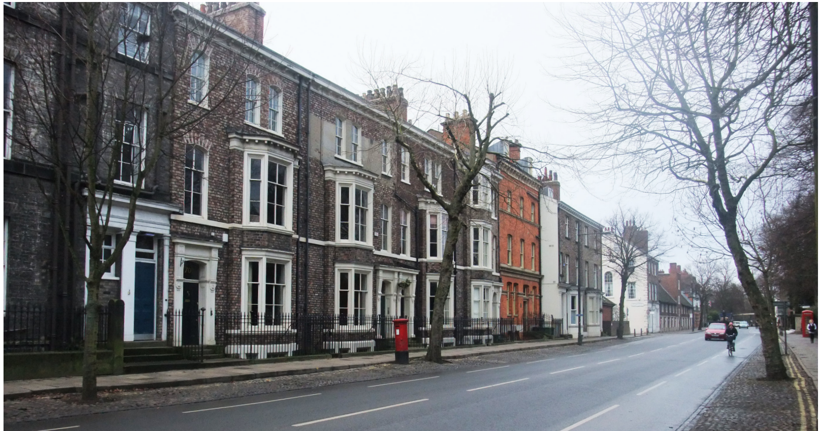
Bootham is wide enough to accommodate traffic, cyclists and pedestrians
