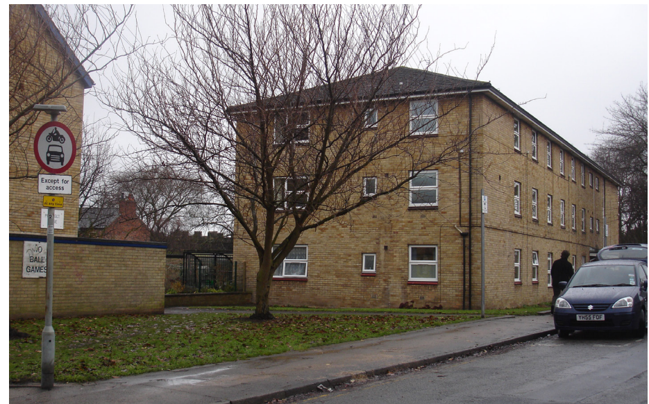
An inappropriate housing block amongst terraced streets
