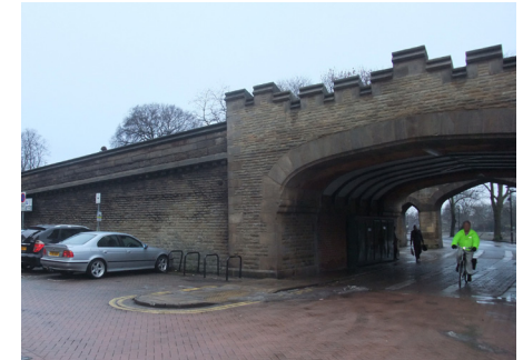
Space along the riverside walk can be better utilised. At present the area along Tanners Moat is used for a surface level car park
