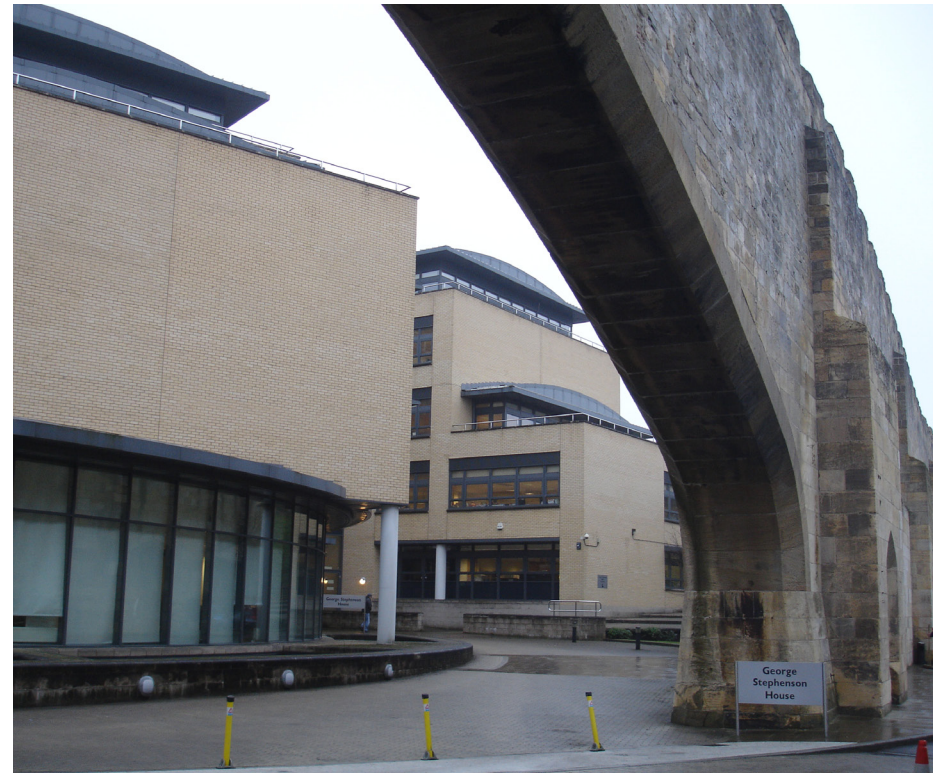
The rooftop points of George Stephenson House are higher than the walls
