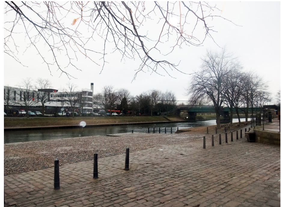
The Royal Mail building is highly visible from the riverside walkway in winter
