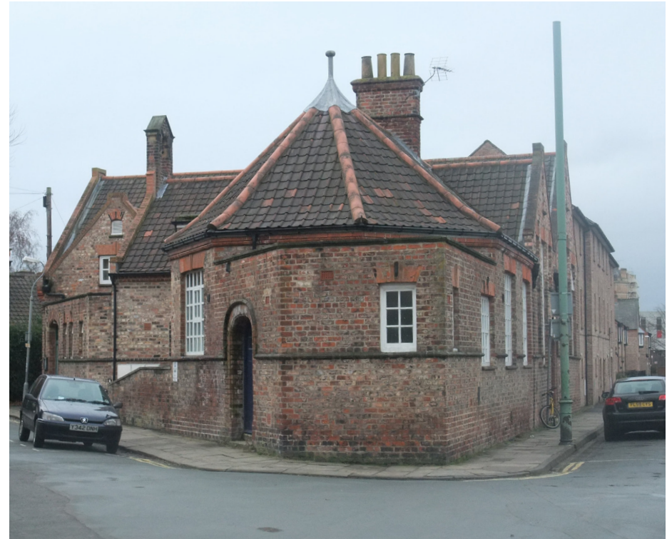
The Sunday School on the corner of Frederic Street, a Building of Merit. It has been converted for residential use.
