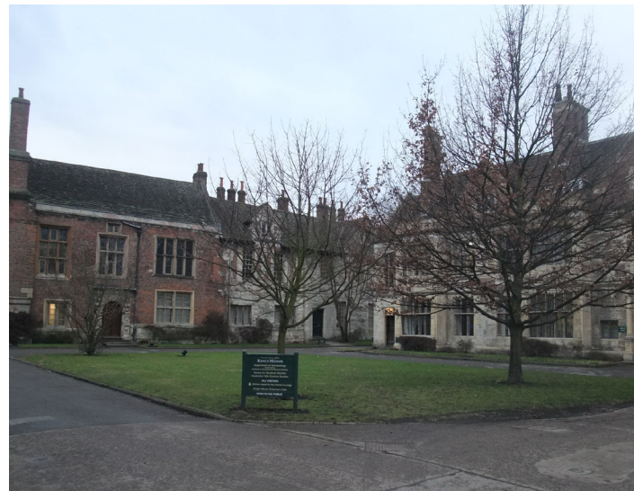
Grade I Listed King's Manor, which dates back to the 15th century (left) and the Victorian Headmaster's House (right)
