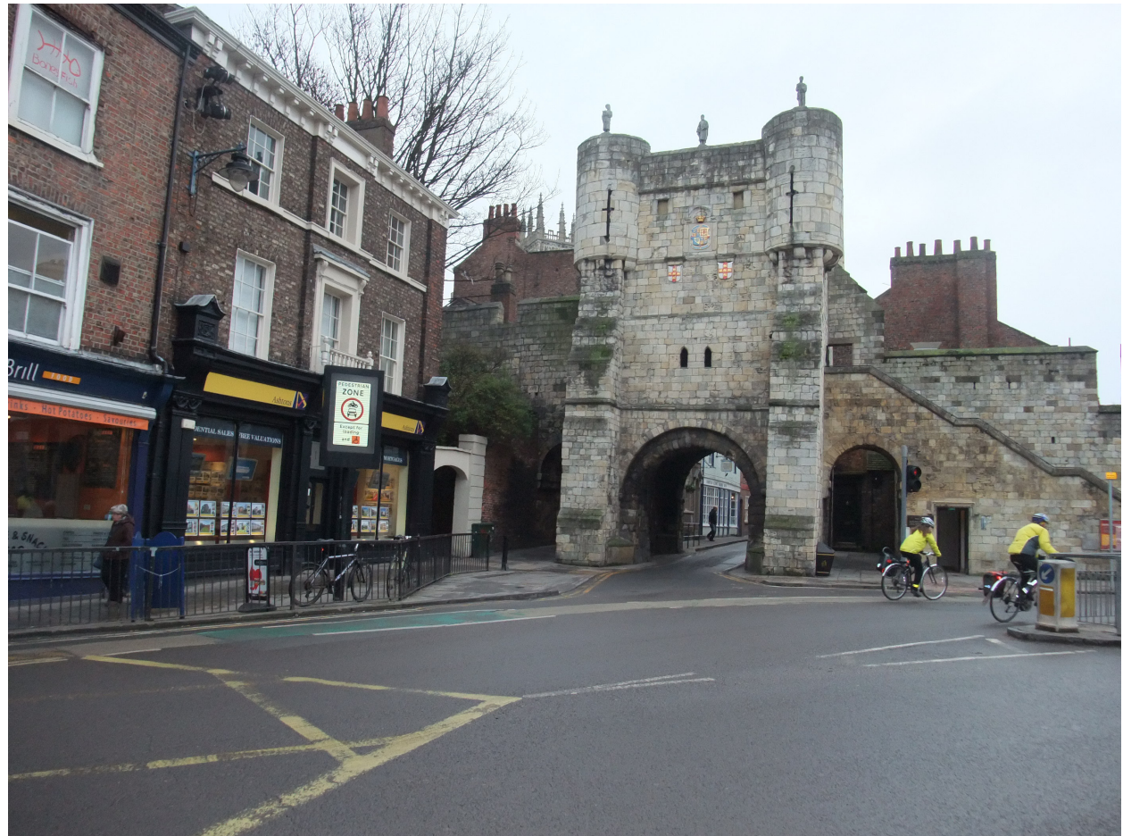
Railings and road markings compromise the setting of Bootham Bar
