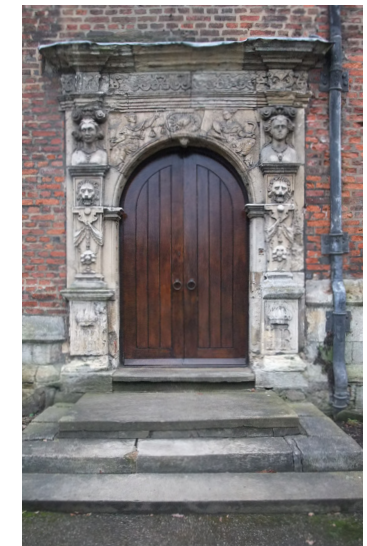
A carved early 17th century doorway at the King's Manor
