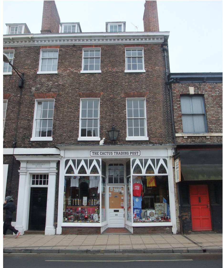
No. 26 Gillygate is Grade II* listed
