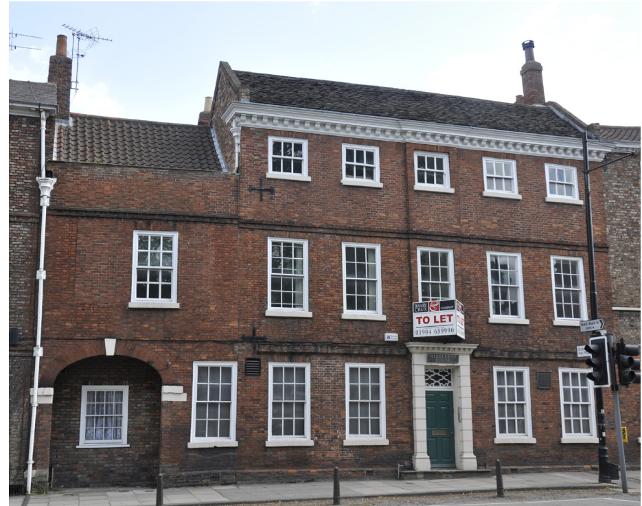
Middleton House (No. 38) is the finest house on the street. The earliest parts date from about 1700 and it was heightened in 1765. It was initially built for a gentleman and then owned by a baker and a silkweaver. In 1798 the house was bought by Rev. Charles Wellbeloved who became the principal of Manchester College.
