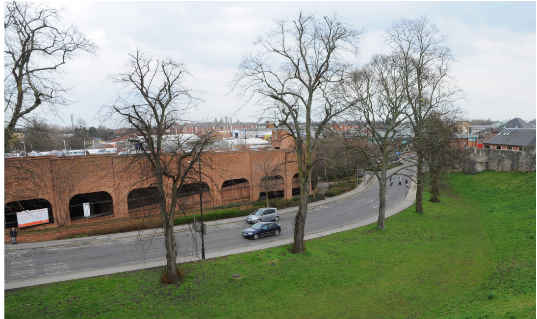
The ramparts along Jewbury are lined with semi mature trees
