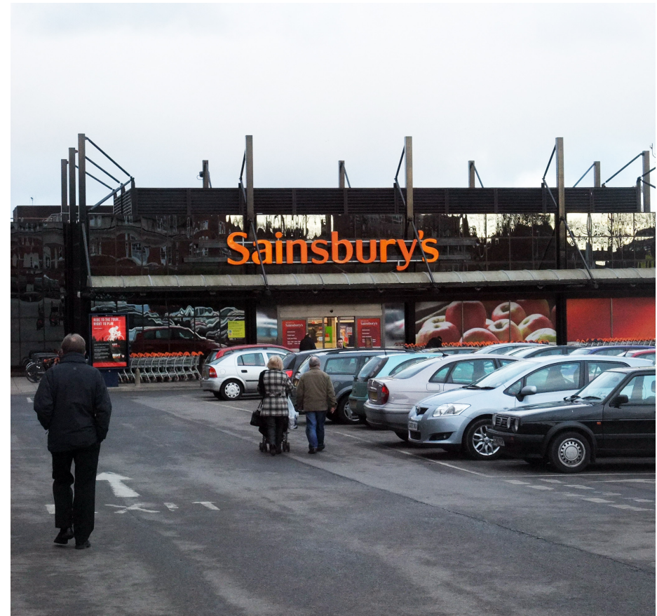
The "big box" retail unit Sainsbury's has been omitted from the Conservation Area as it is not of any special architectural or historic interest
