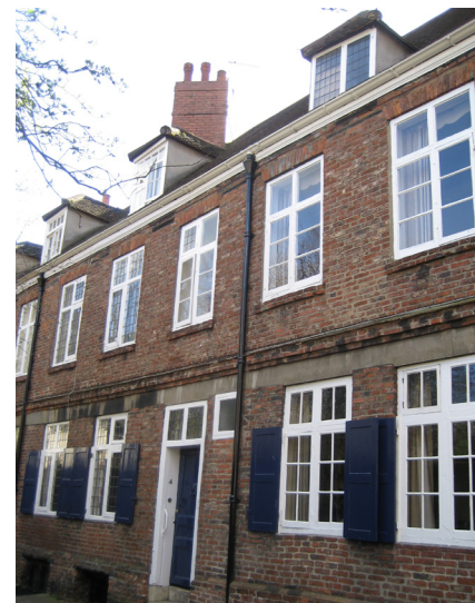
Surviving casement windows in Precentors Court
