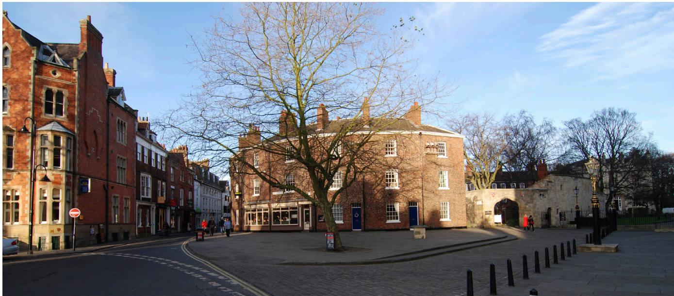
The public space at the west end of The Minster was created in phases in the 19th century by demolishing houses and shops
