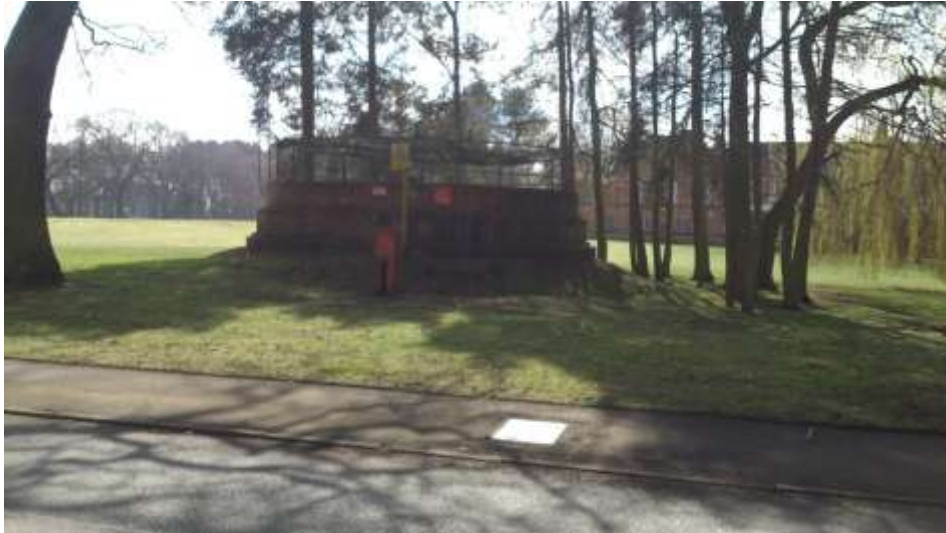
Photograph 1: Southeast facing photograph of water tank (building 82). The development area is within the background.
