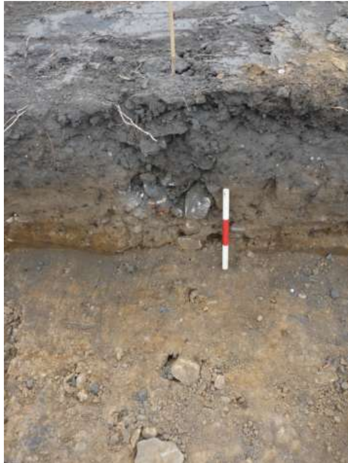
Plate 32 Context 2302 facing south, scale unit 0.1m
