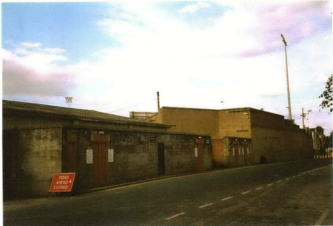
Plate 3. Bootham Crescent Football Ground Offices and Turnstiles fronting Grosvenor Road. Facing north-east.
