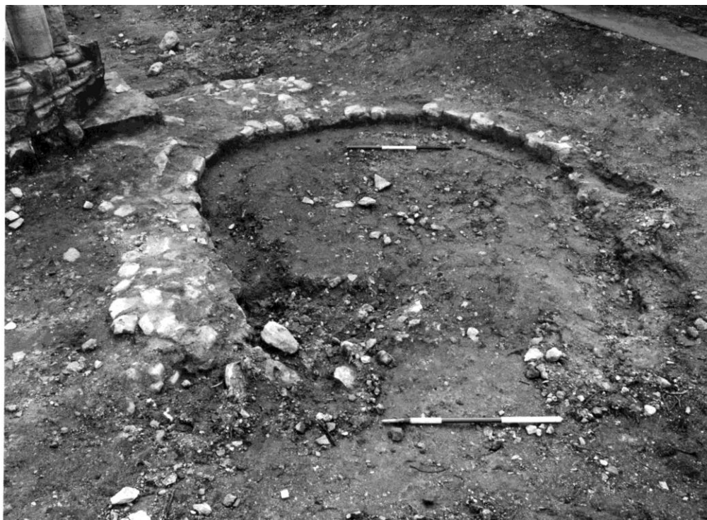
Figure 11: Photograph, looking NE, of consolidation works on the north transept in advance of planning out of the Abbey. Photo by RCHME in the archive of the Yorkshire Museum.
