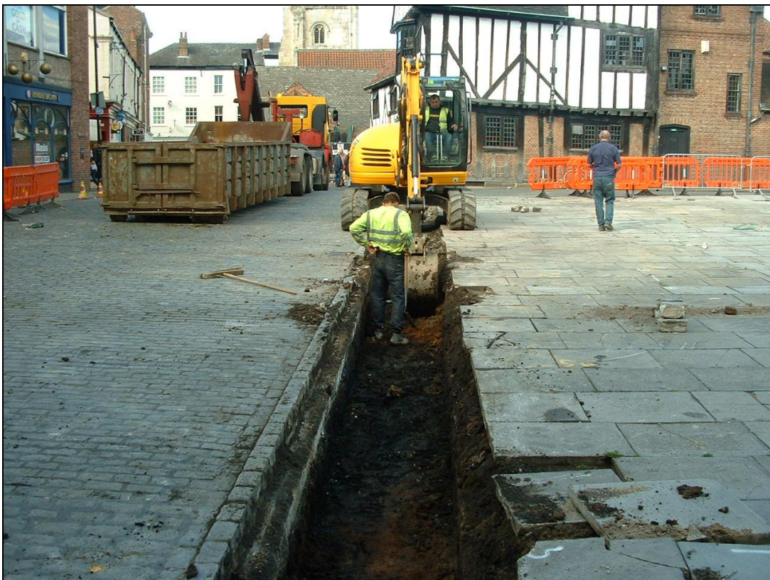
Plate 22. Area 4 under excavation, looking NW
