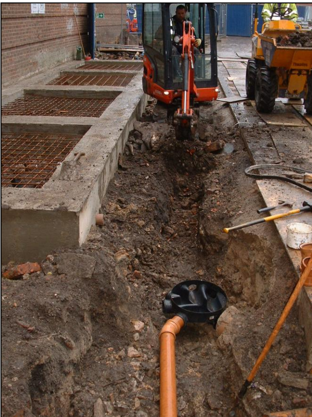
Plate 24. Area 6 under excavation, looking NW
