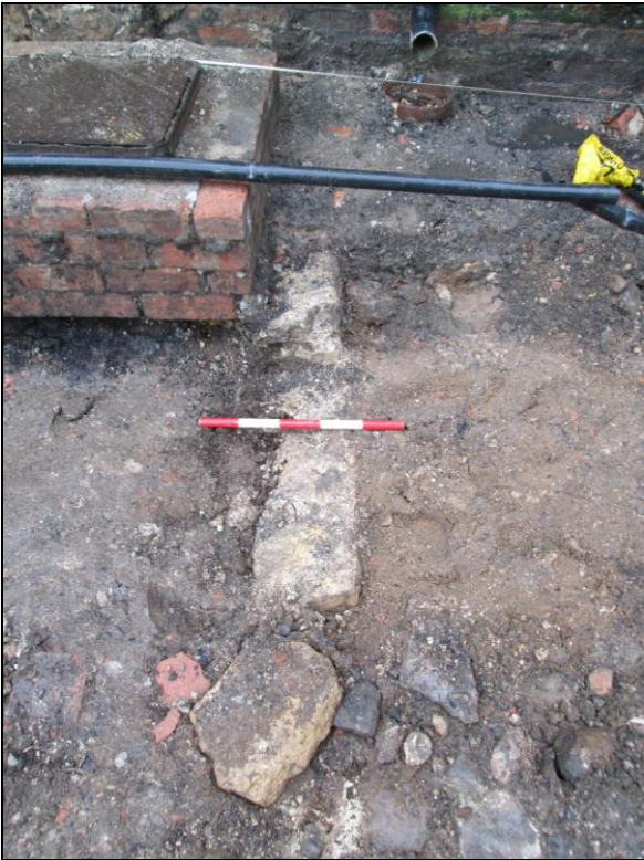
Plate 11. Wall (214), looking NE
