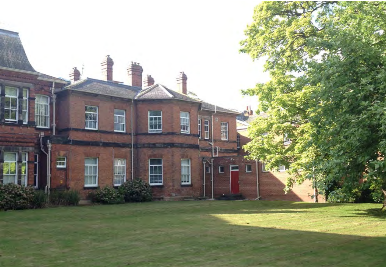
North-east elevation of the Service Block
