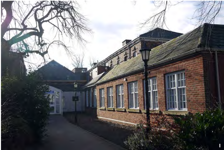
1 The rear entrance of the Hospital and the Elderly Administrative offices to the right, 2015 2 The rear of the wing from the north-west
