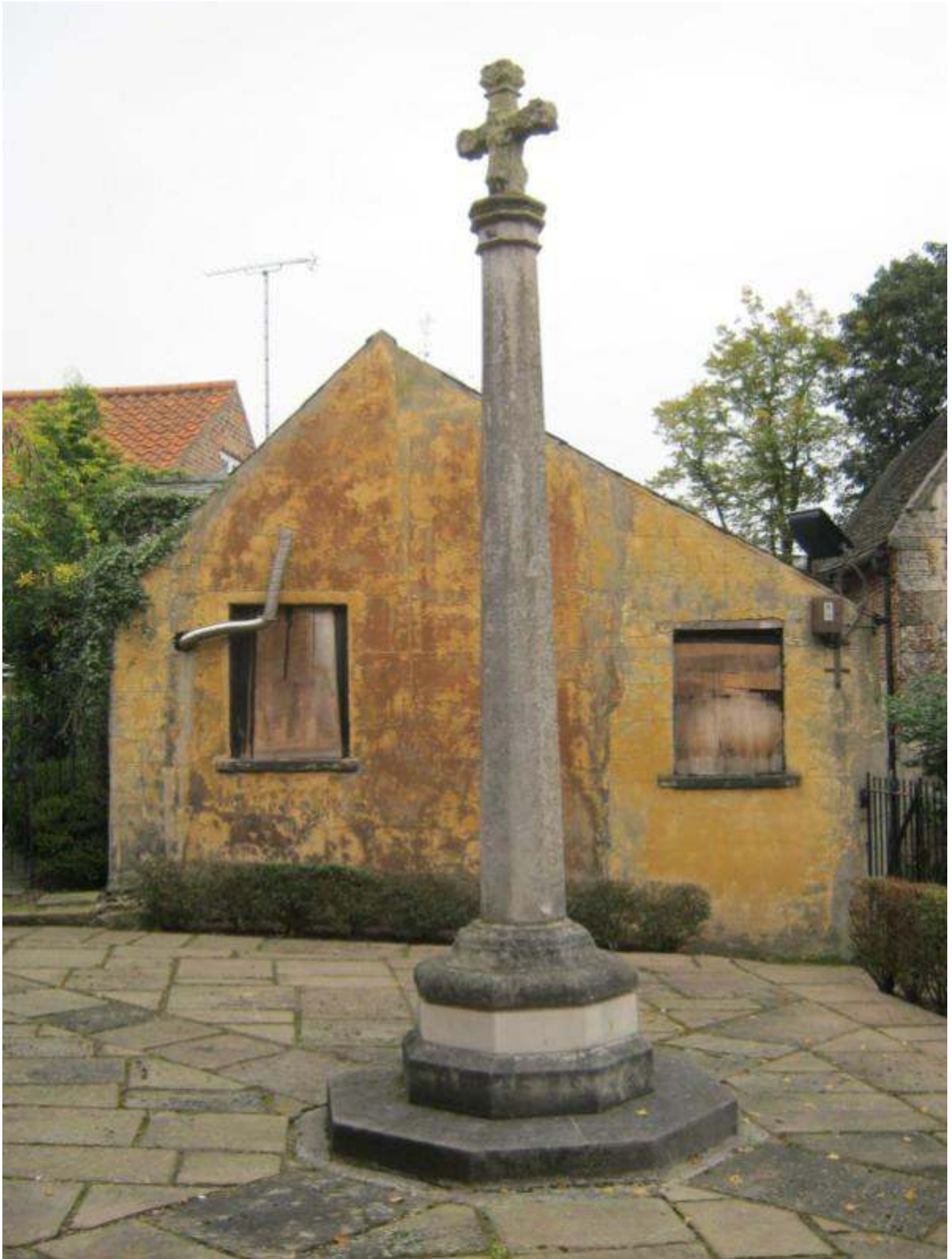
South-west facing facade of the derelict boxing club/former mortuary chapel.
