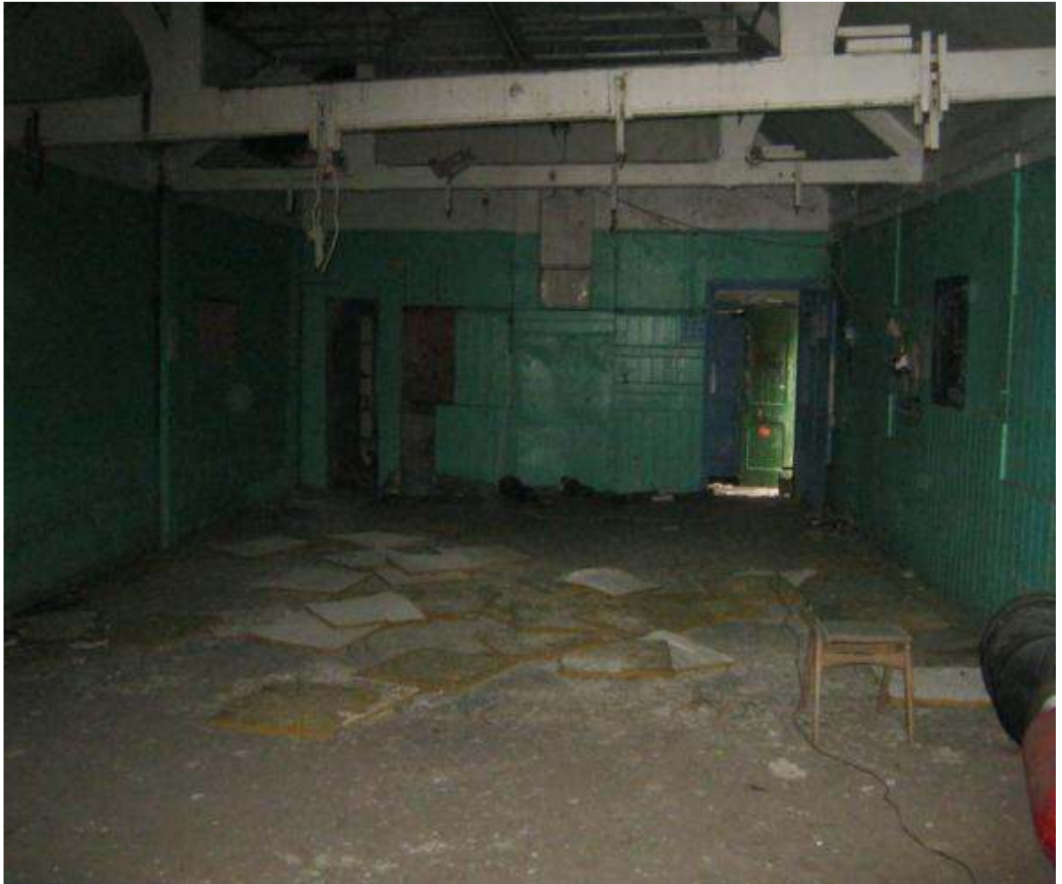
Interior of the derelict boxing club/former mortuary chapel.
