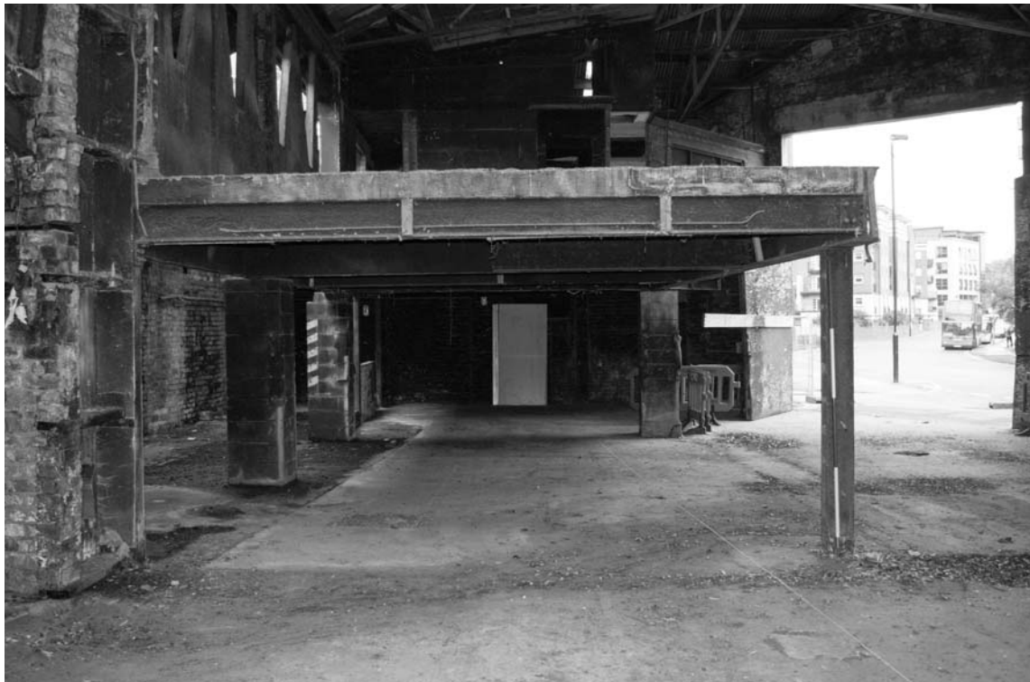
Photograph 70. The mezzanine's steel structure
