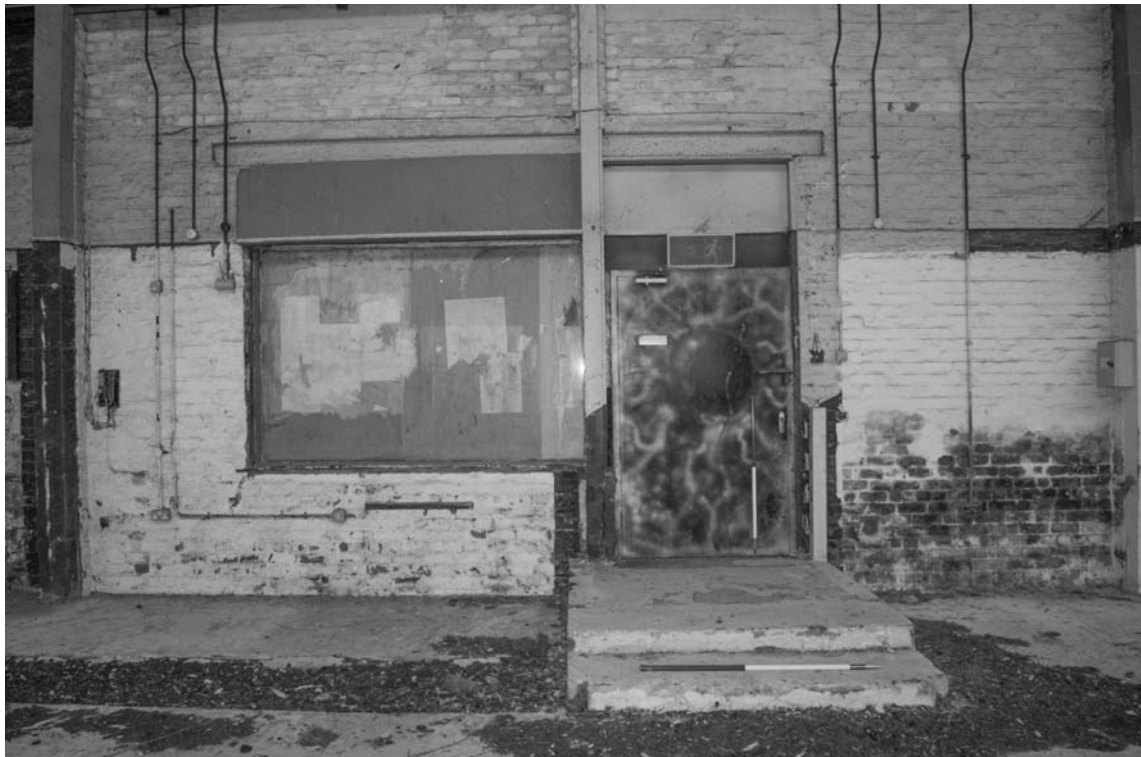
Photograph 58. A later inserted door and window with concrete steps up. Note the steel lintel
