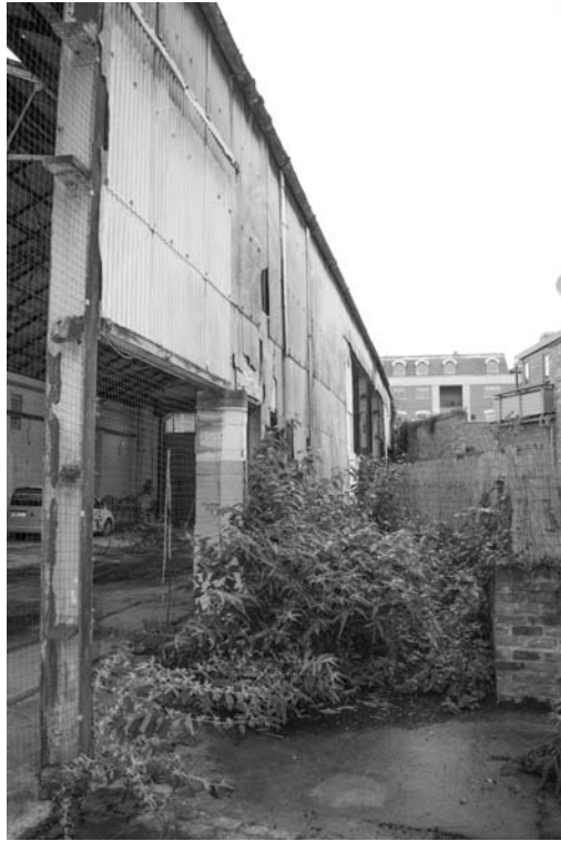
Photograph 29. The rear of the building with panels missing at low level
