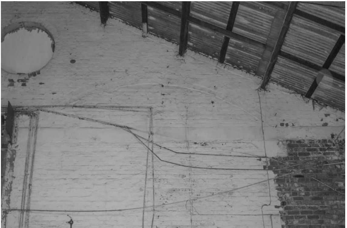
Photograph 52. A brick segmental relieving arch
