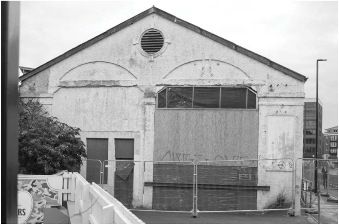
Photograph 21. The north gable end of 17-21 Piccadilly with perspective control
