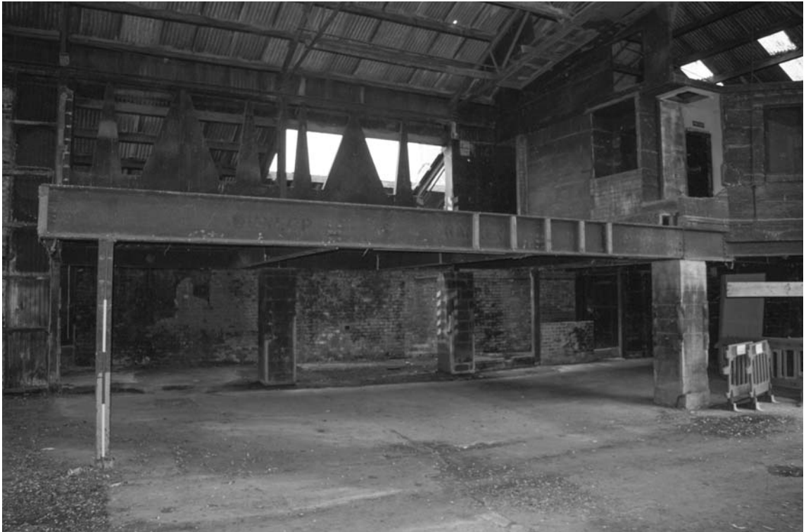
Photograph 71. The mezzanine's steel structure
