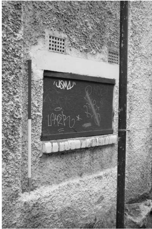
Photograph 33. A small window, possibly inserted with bull-nosed brick sill
