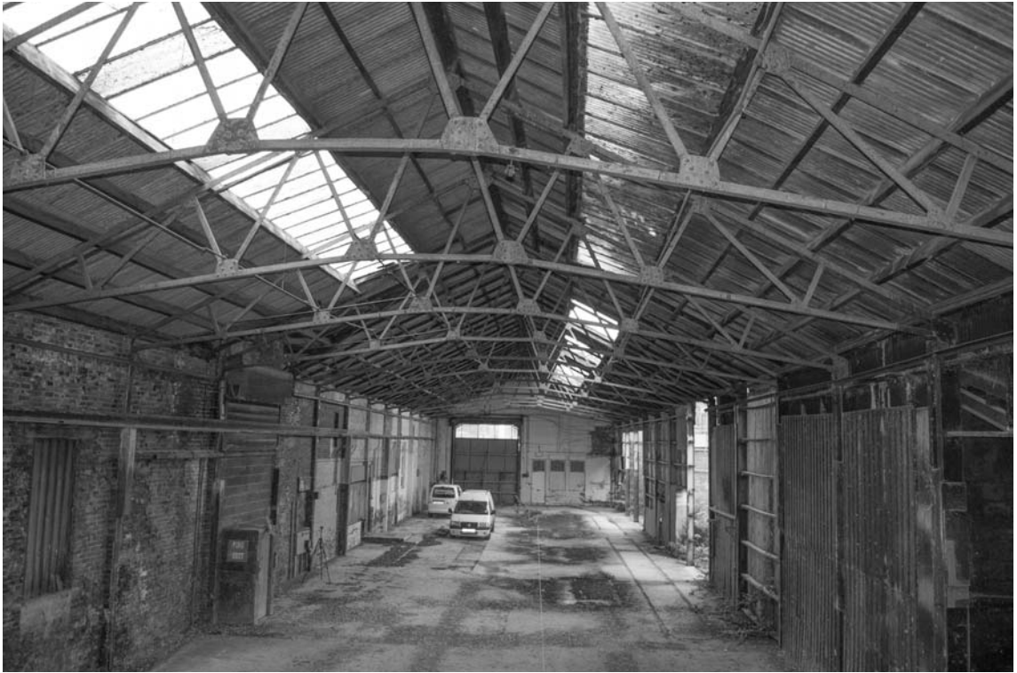
Photograph 41. View of interior showing steel roof trusses
