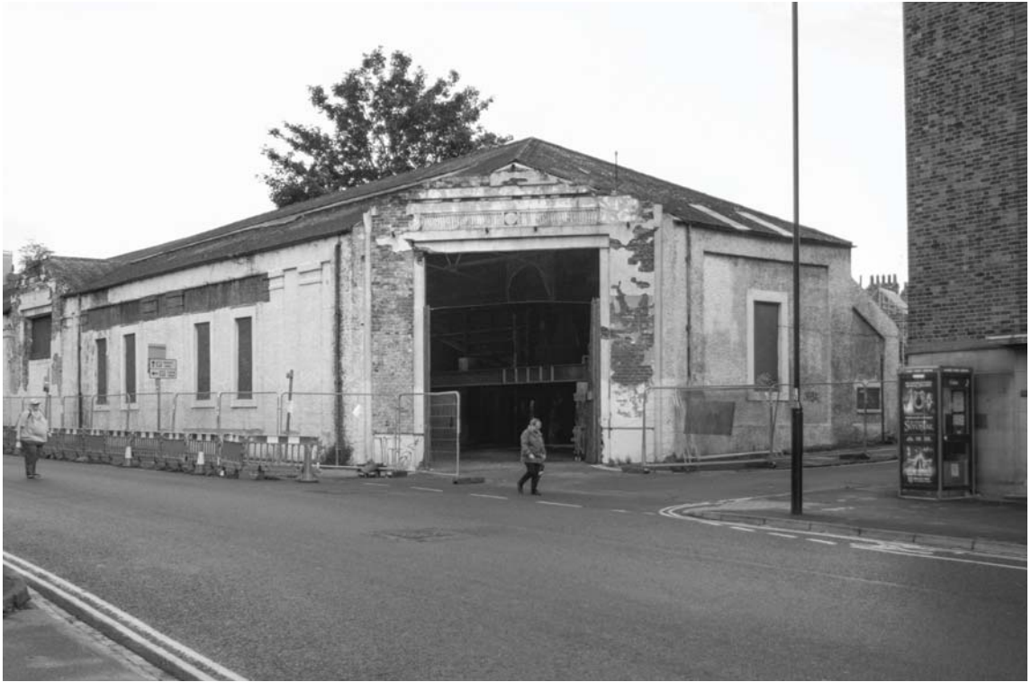
Photograph 3. View of the southern chamfered or canted gable
