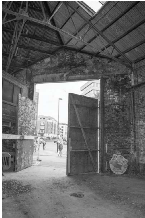
Photograph 61. The interior face of the chamfered or canted gable
