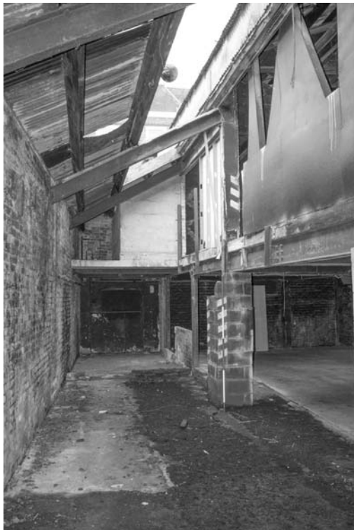
Photograph 74. Interior of the lean-to with mezzanine toilet above
