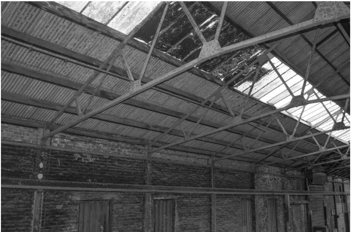
Photograph 42. Detail of trusses bolting to steel stanchions
