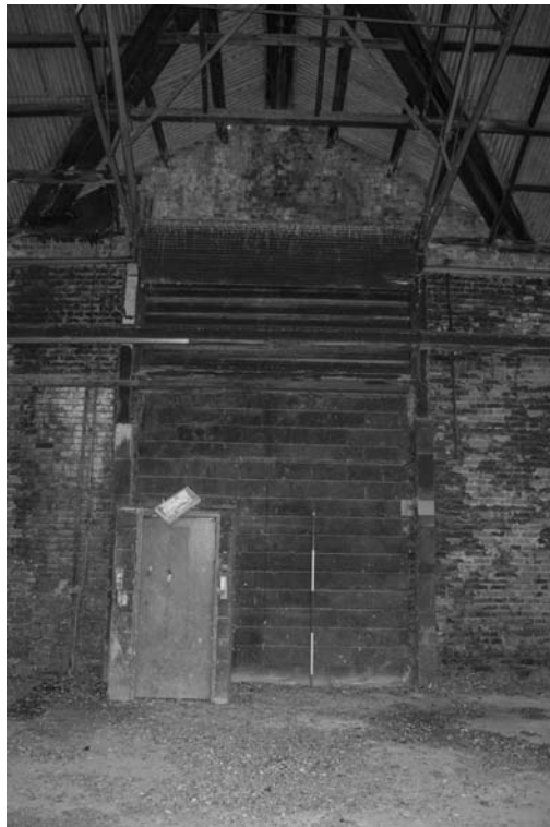
Photograph 59. A breeze-blocked entrance in the gablet with incorporated vestibule and door
