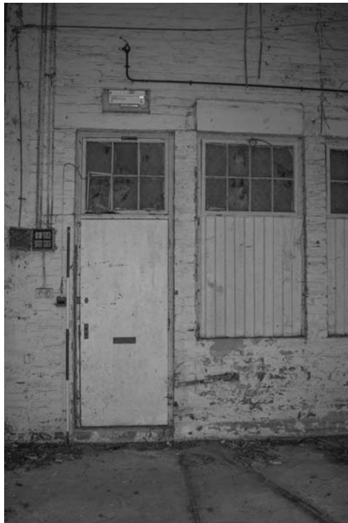
Photograph 46. Doorway and window in the north gable
