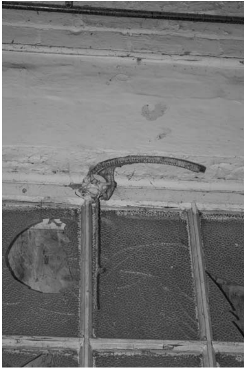
Photograph 47. A cogged window opener
