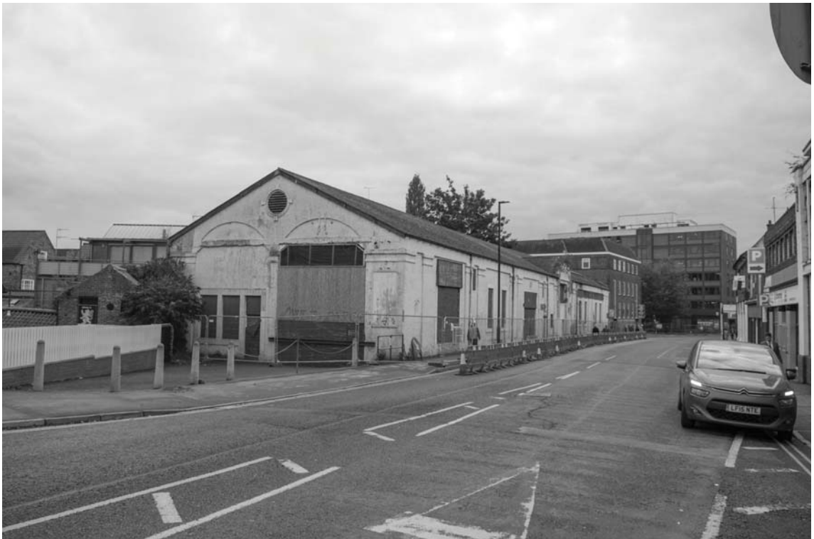
Photograph 17. General view south along Piccadilly to no. 17-21
