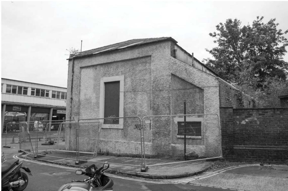
Photograph 31. Part of the south elevation with central window and lean-to
