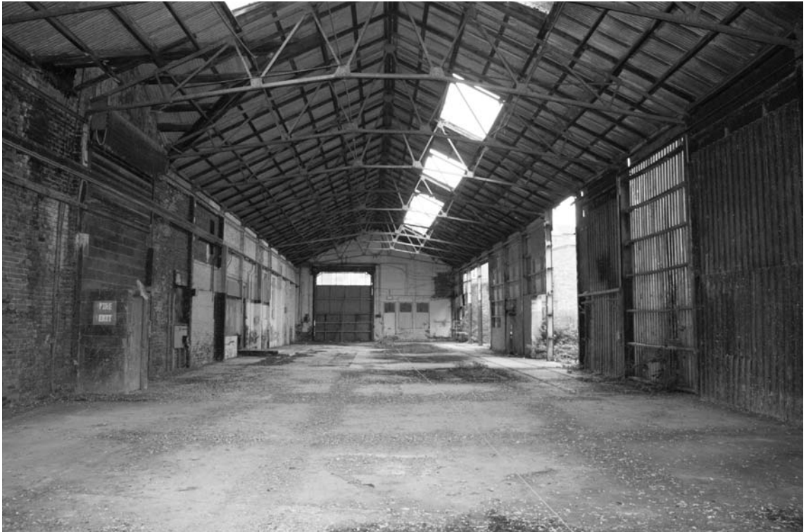
Photograph 35. General view of the interior to the north gable
