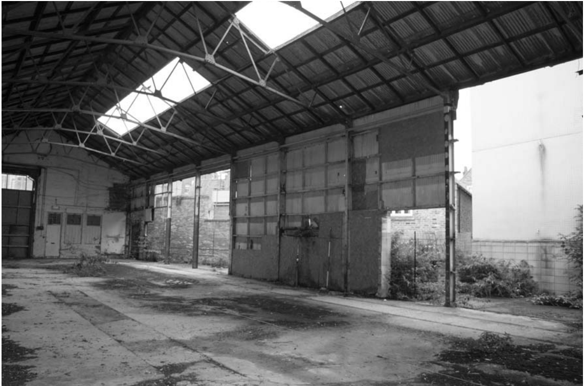
Photograph 37. General view of the rear elevation interior
