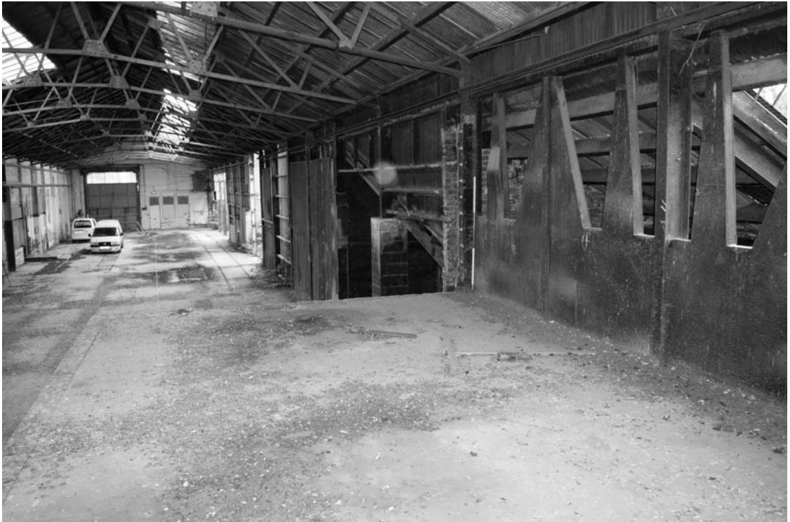
Photograph 77. The open concrete platform makes up most of the mezzanine
