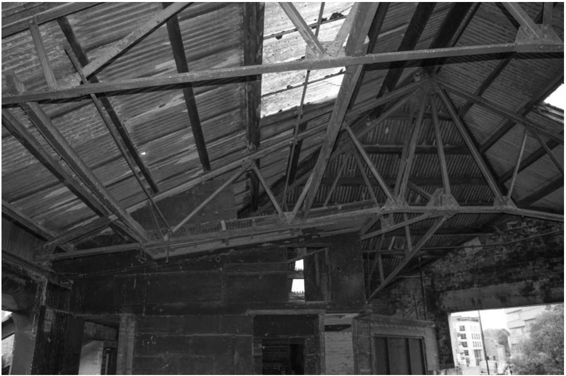
Photograph 85. The storage area above the mezzanine offices
