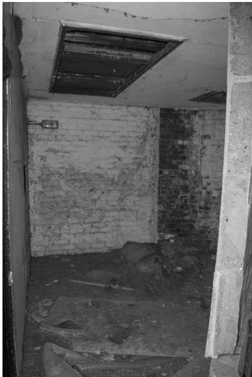
Photograph 82. The interior of room M4 with access to roof storage
