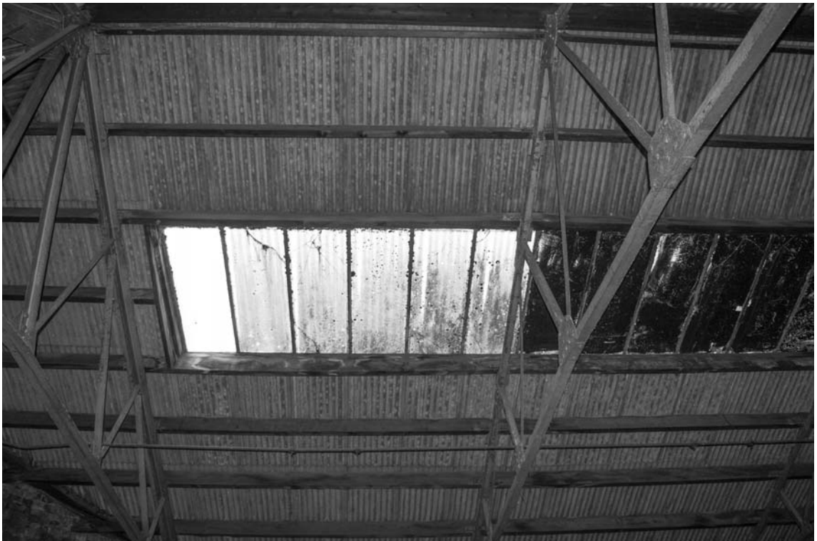
Photograph 43. Detail of a rooflight
