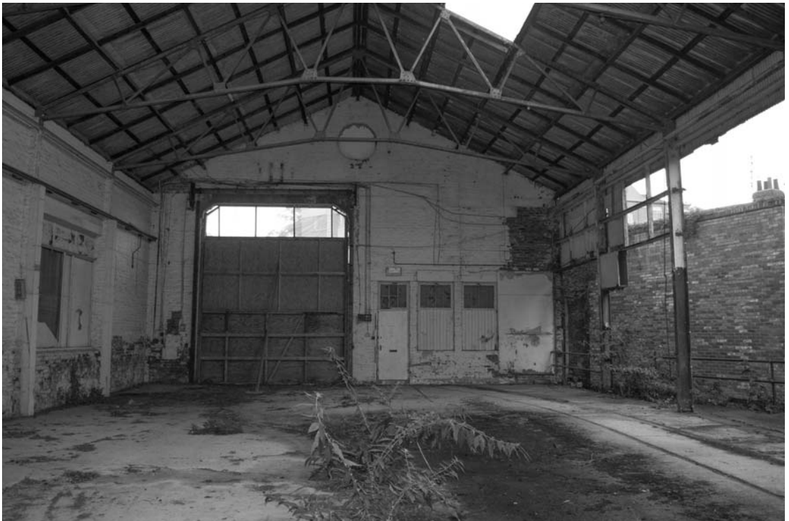
Photograph 44. The north gable interior
