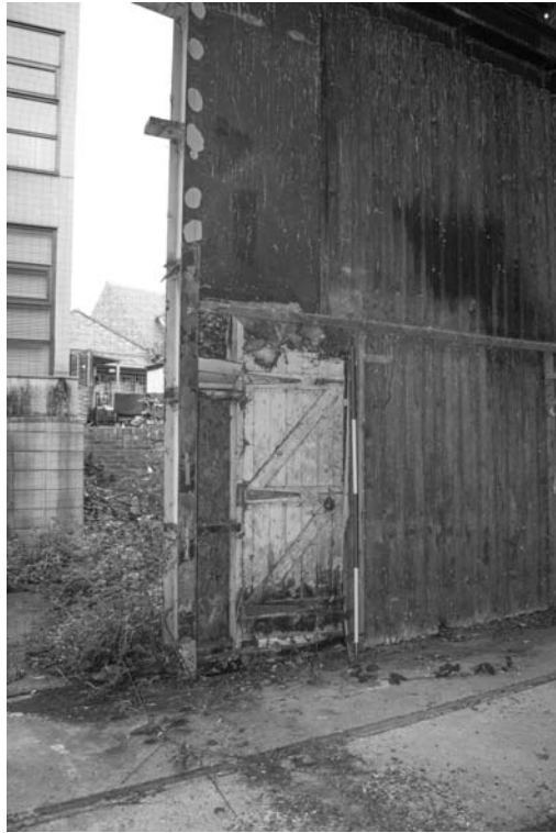
Photograph 65. A batten door out to a rear courtyard
