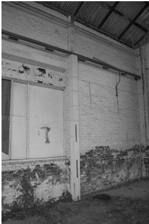
Photograph 54. Modern breeze block built up against the steel stanchion and brick
