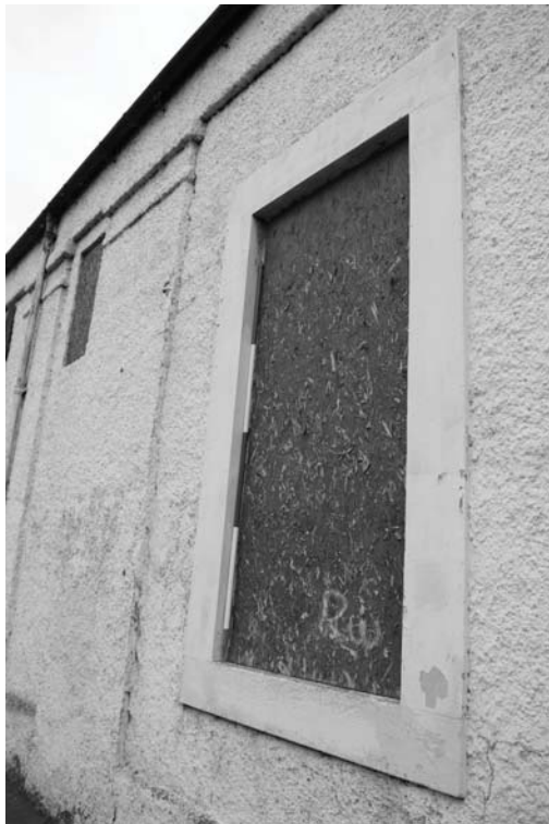
Photograph 12. A typical external window surround
