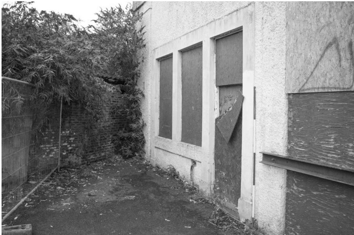
Photograph 26. Doorway and windows in blocked-up entrance
