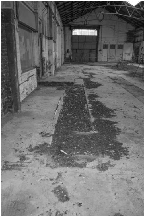
Photograph 68. A possible concrete-filled vehicle inspection pit
