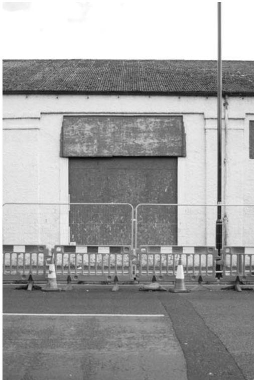
Photograph 10. The boarded-up modern window in external bay 7 with perspective control
