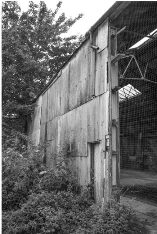
Photograph 30. The rear elevation with a small doorway in the asbestos cladding
