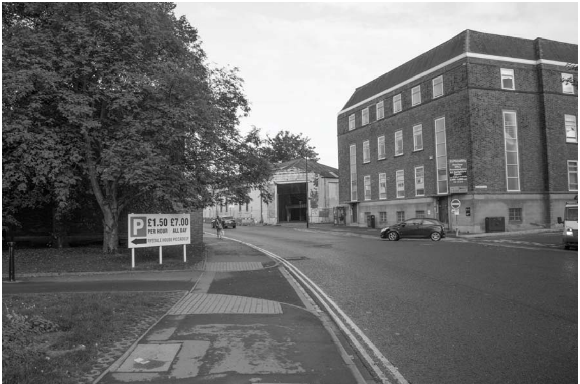
Photograph 1. General view north along Piccadilly to no. 17-21
