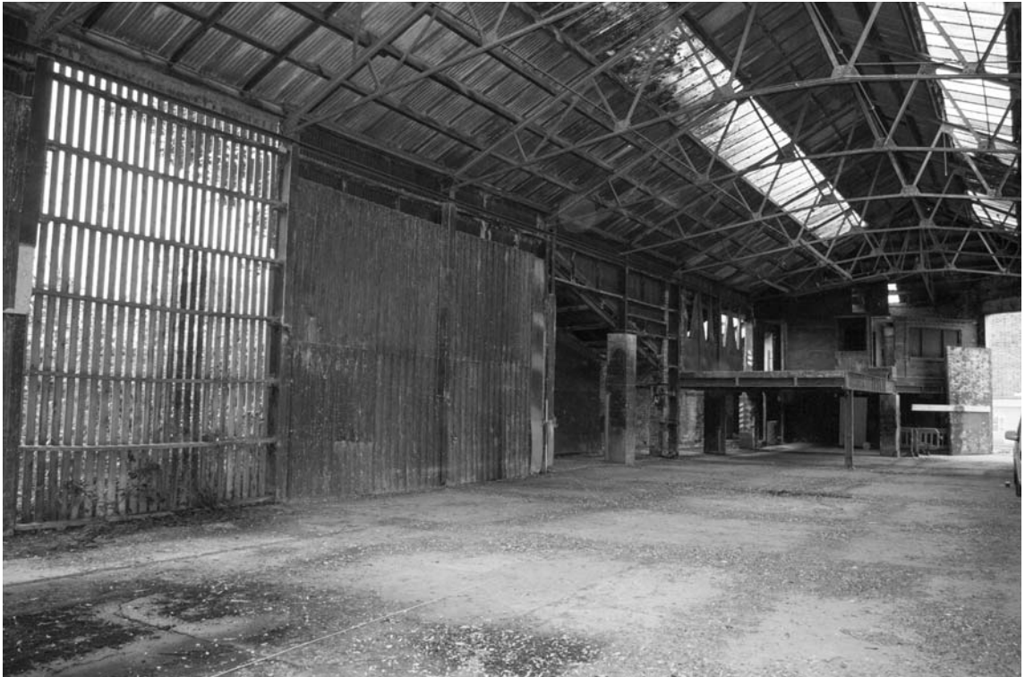
Photograph 39. General view showing timber frame with corrugated cladding
