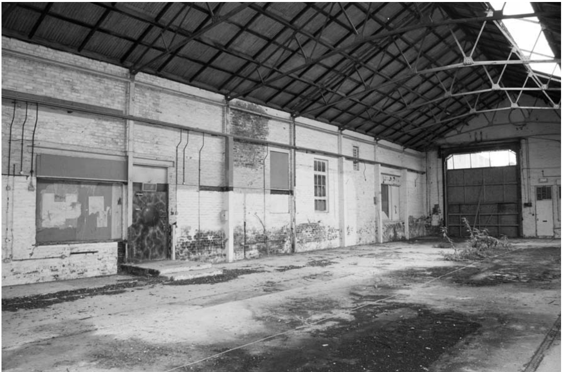
Photograph 38. General view of the front elevation interior
