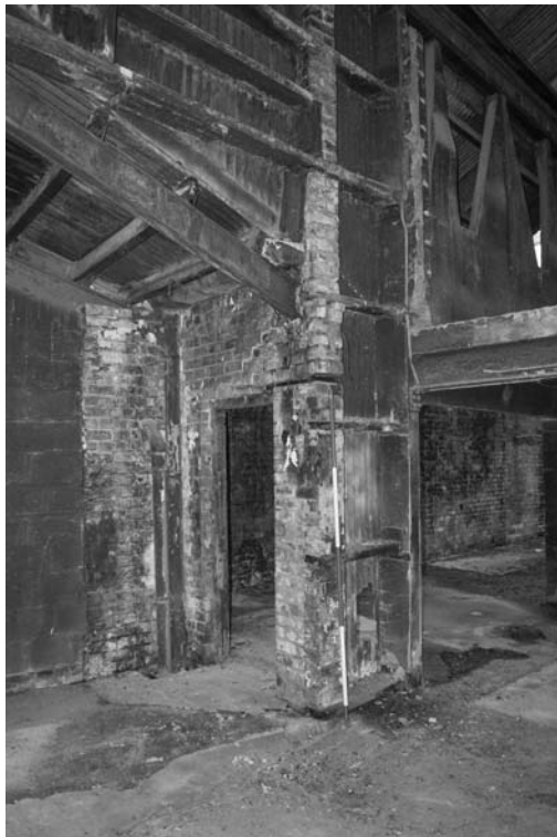
Photograph 76. An area where brickwork meets timber frame
