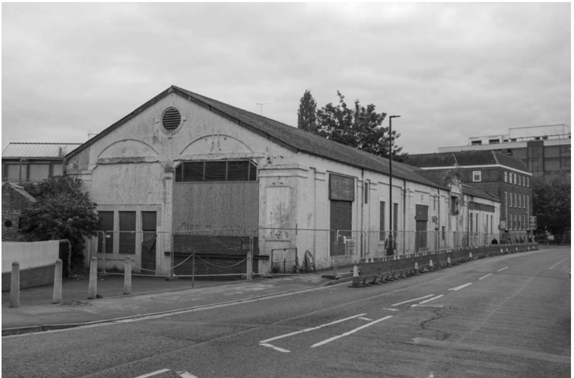
Photograph 18. General view of no. 17-21 Piccadilly
