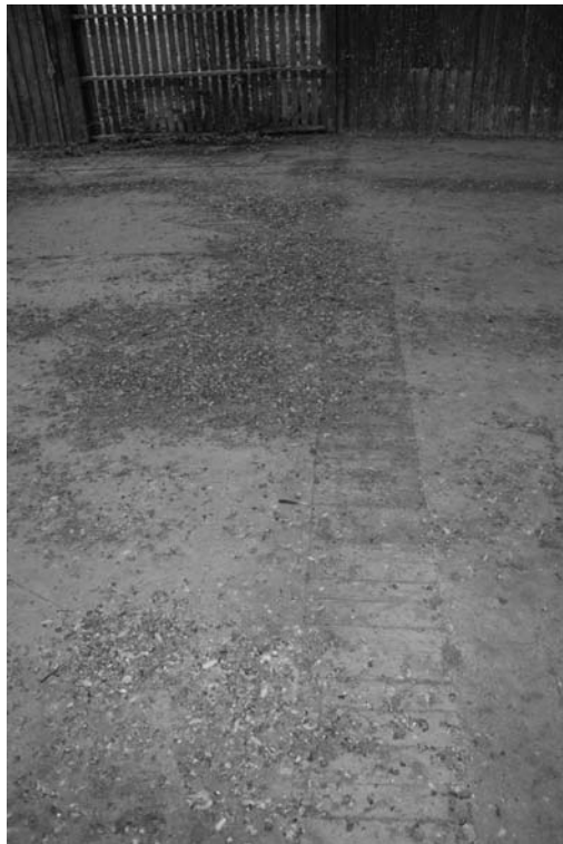
Photograph 69. Short timber boards providing access to a service trench
