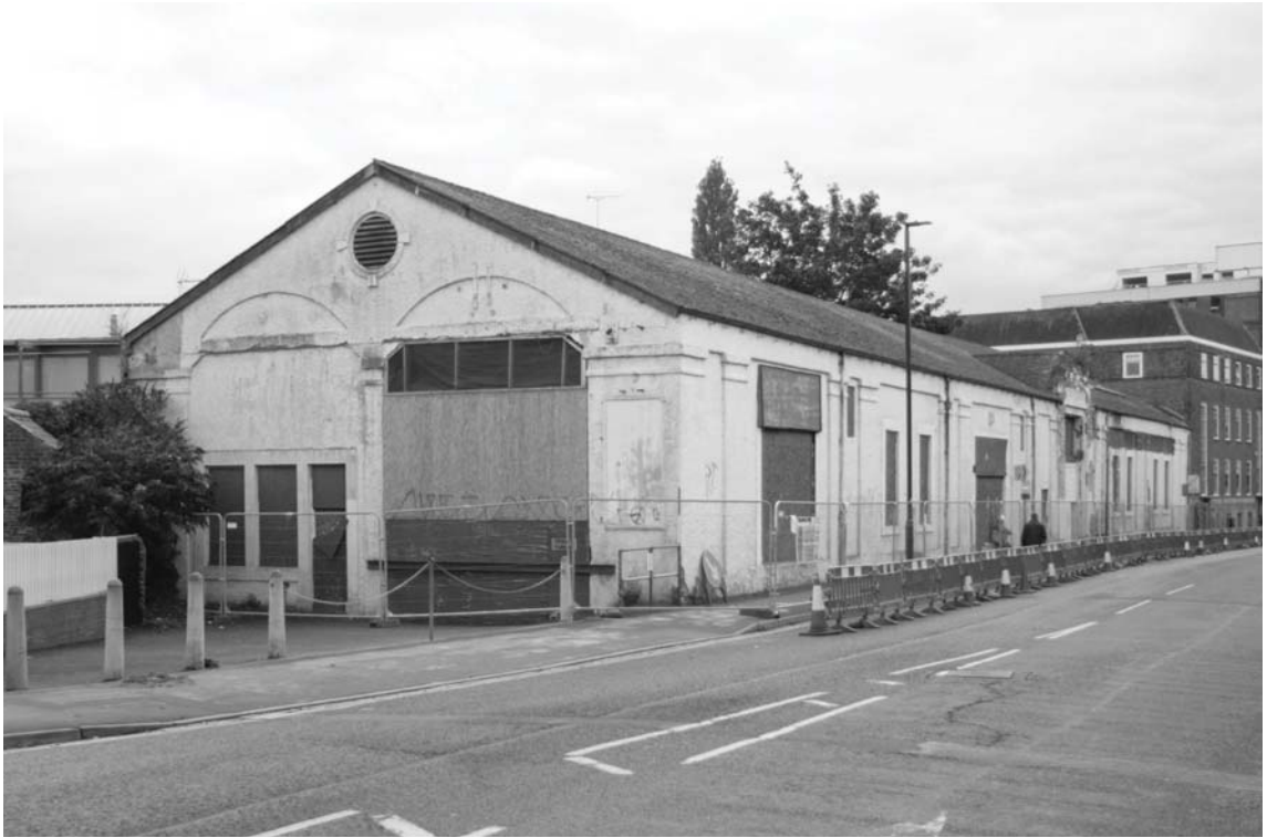
Photograph 19. General view of no. 17-21 Piccadilly with perspective control
