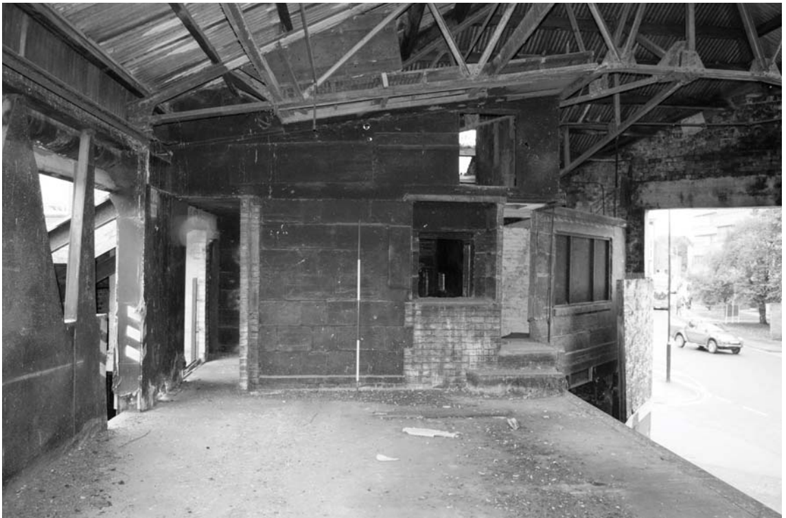
Photograph 78. The offices with breeze-block built around brick
