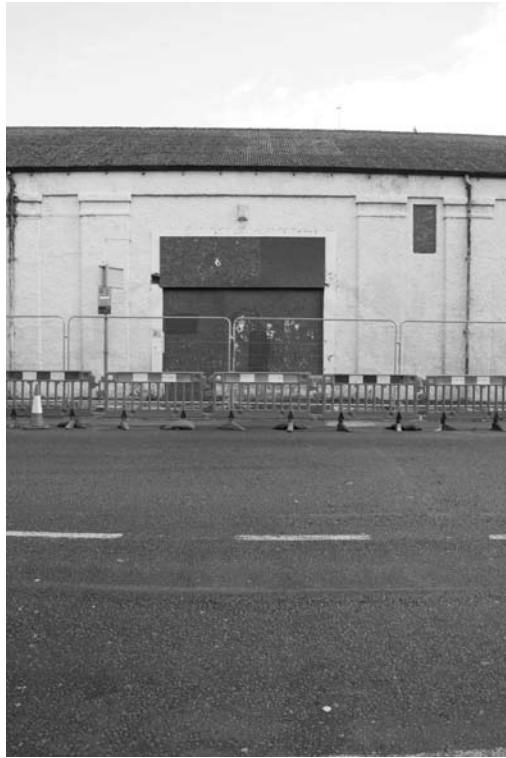
Photograph 7. The boarded-up door and window in external bay 5
