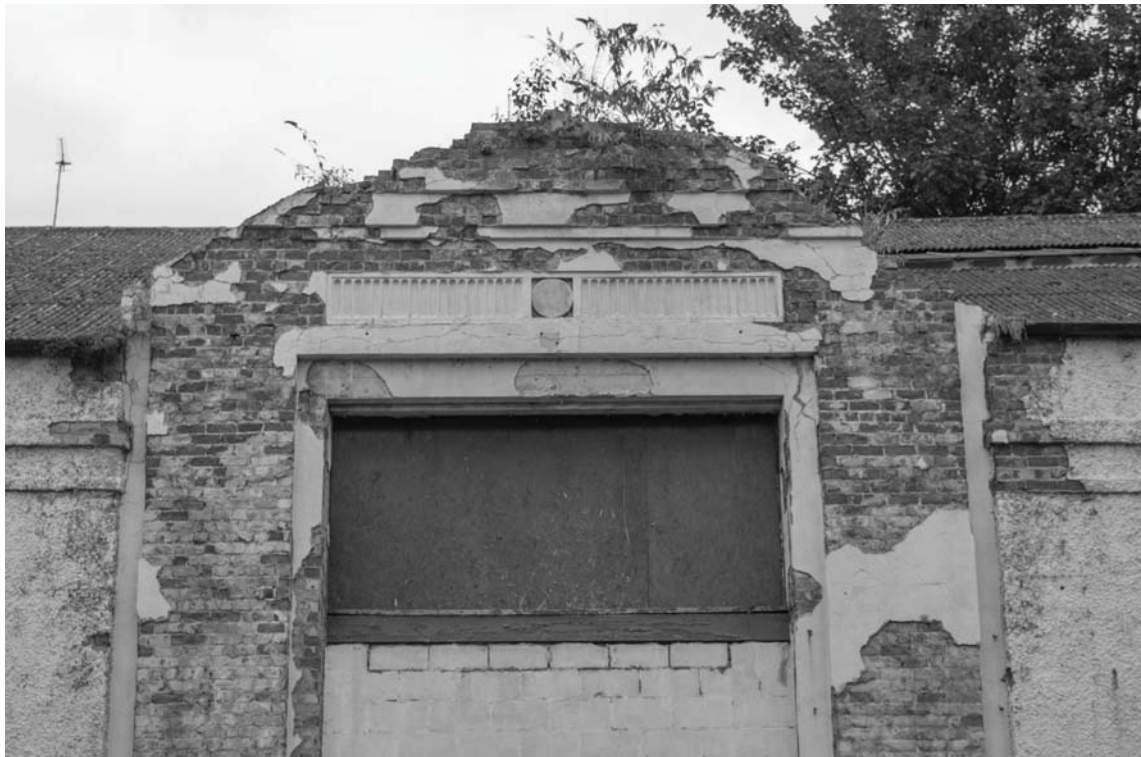
Photograph 14. Detail of the gablet frieze and stepping towards apex
