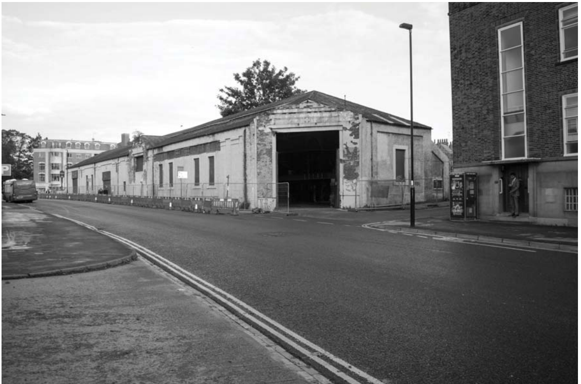
Photograph 2. General view of 17-21 Piccadilly
