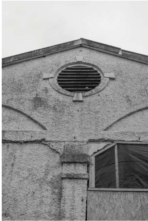
Photograph 23. Detail of moulded corbels with louvered, keyed oculus above
