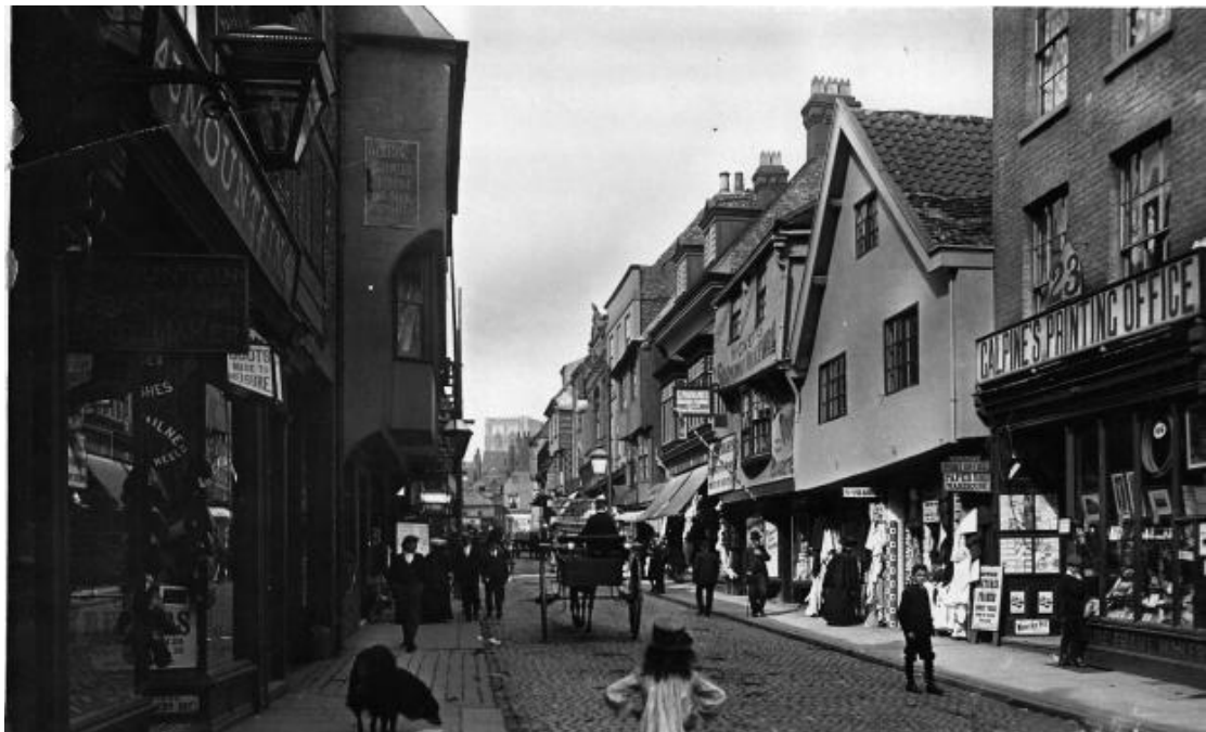
Fig 4: The street frontage before 1911
