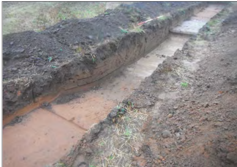
Plate 3. Trench 6, possible quarry pit 604, looking south-east
