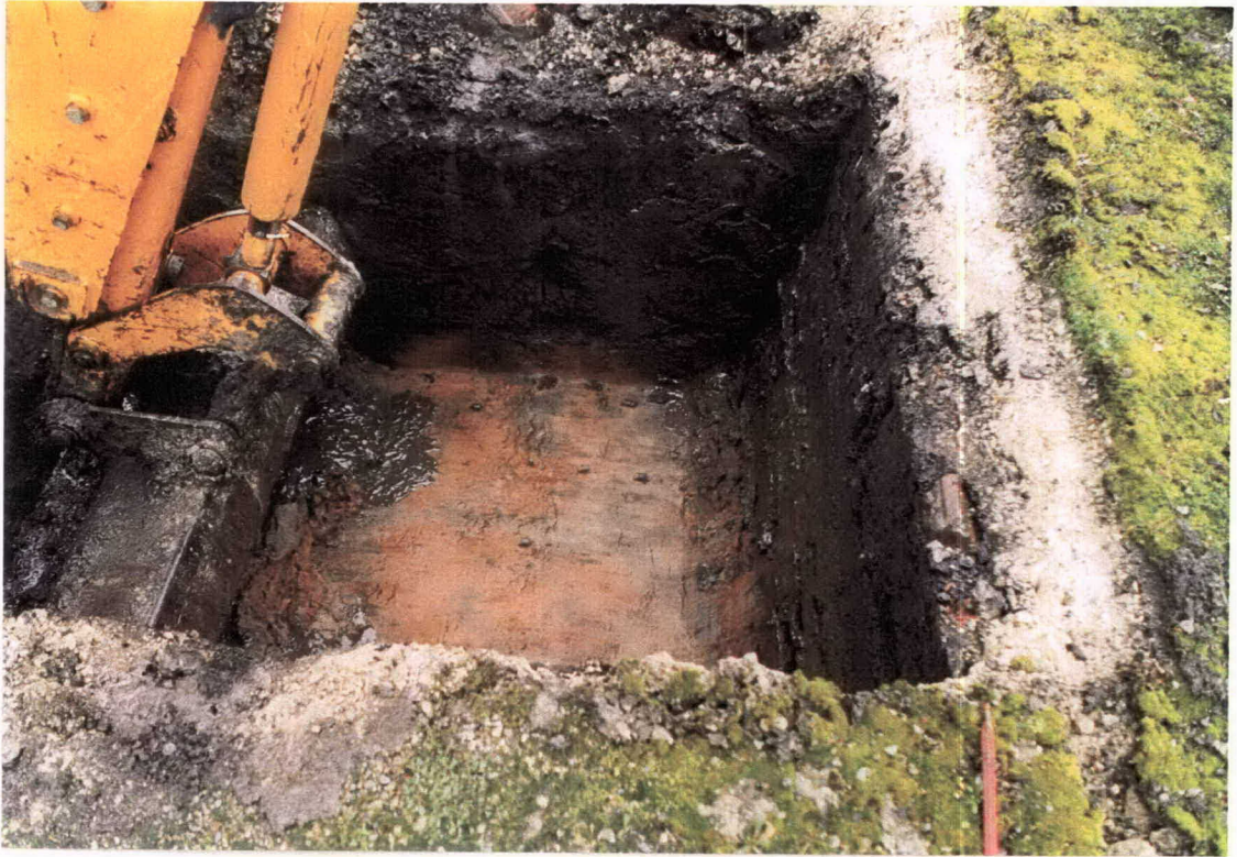
Plate 9. Trench 2. During Excavation. Facing North.
