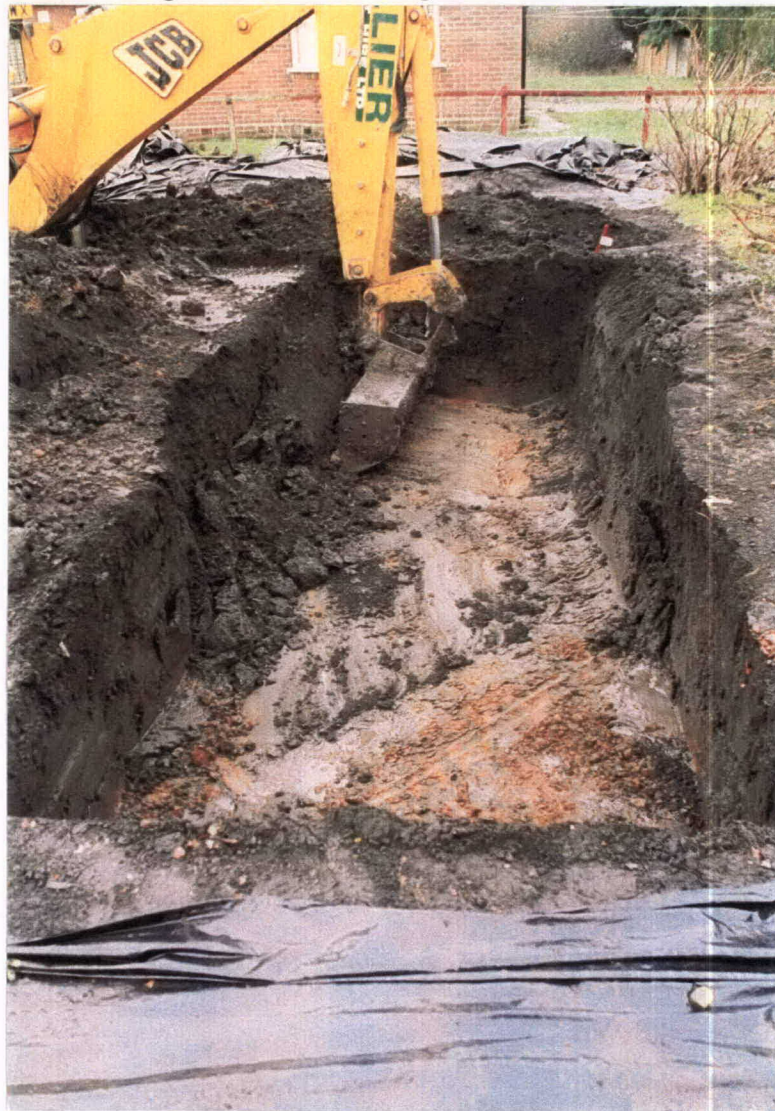
Plate 10. Trench 3. During Excavation. Facing West
