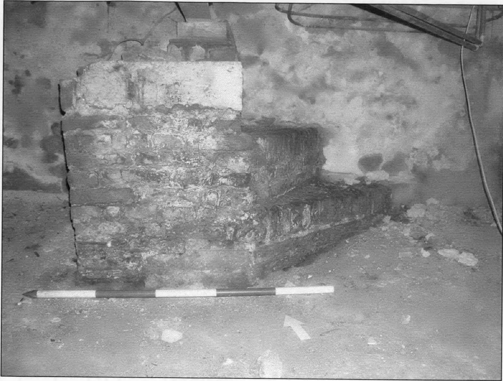
Plate 11 The Old Manor, Clifton: 17th century cellar steps
