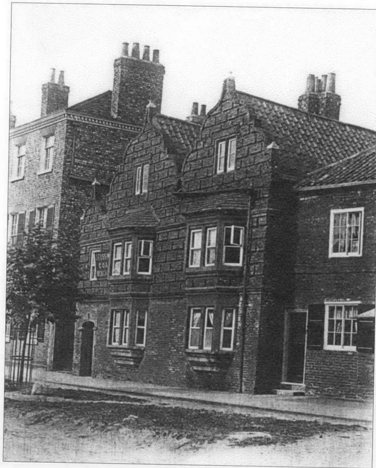
Figure 13 The Old Manor, Clifton: photograph taken c.1895 when John Coussins, coal merchant occupied no. 66
