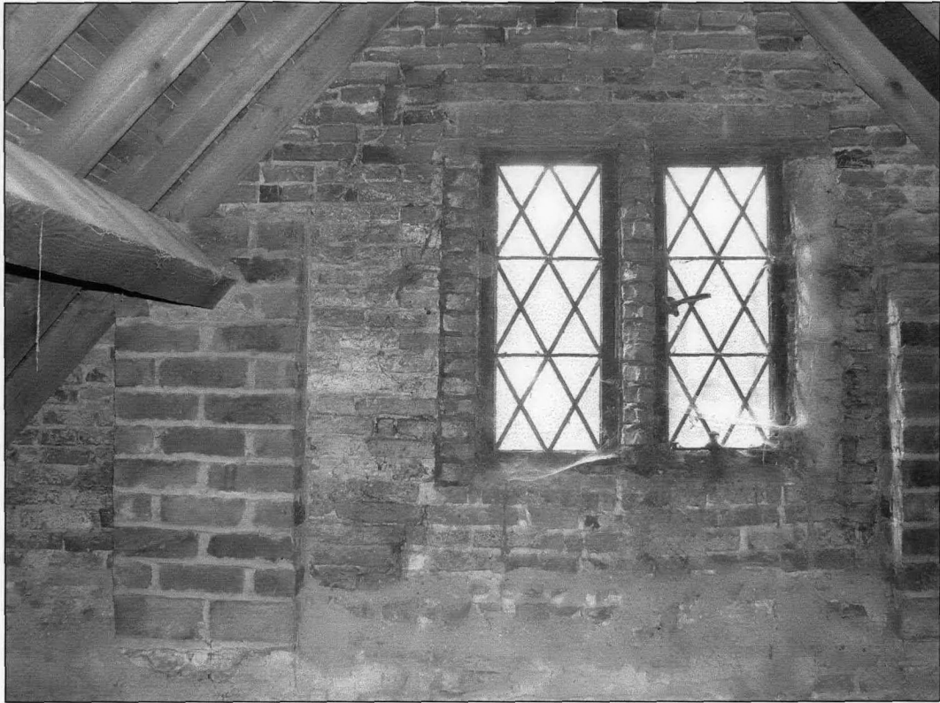
Plate 13 The Old Manor, Clifton: gable window (NW side) showing moulded brick mullions and plaster work concealing void over oriel. Brick pier on left hand side of frame carries modern roof purlin
