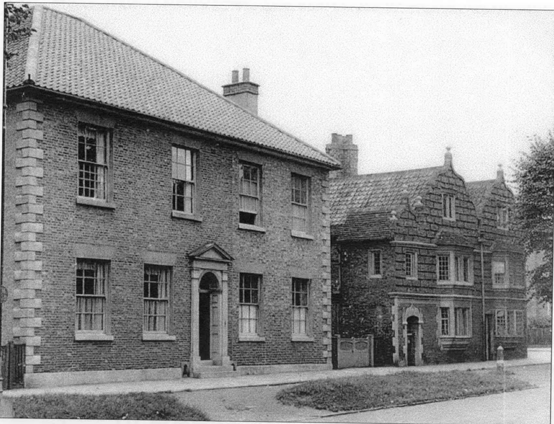
Figure 15 The Old Manor, Clifton: photograph c. mid 1960s after renovations work showing changes to south-east oriel. Clifton Manor in foreground (York City Library)
