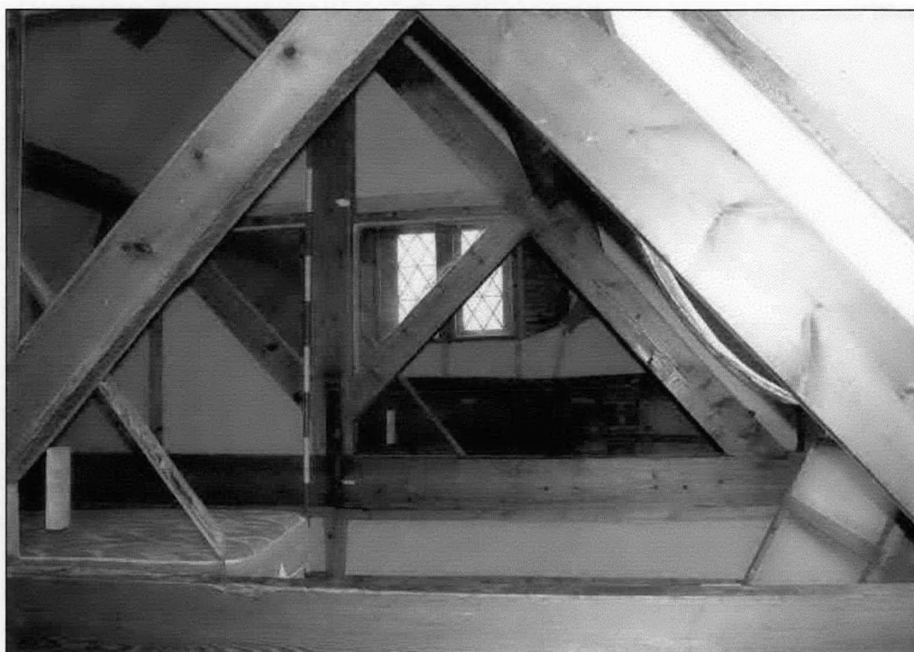
Plate 6 The Old Manor, Clifton: modern roof trusses in no. 64
