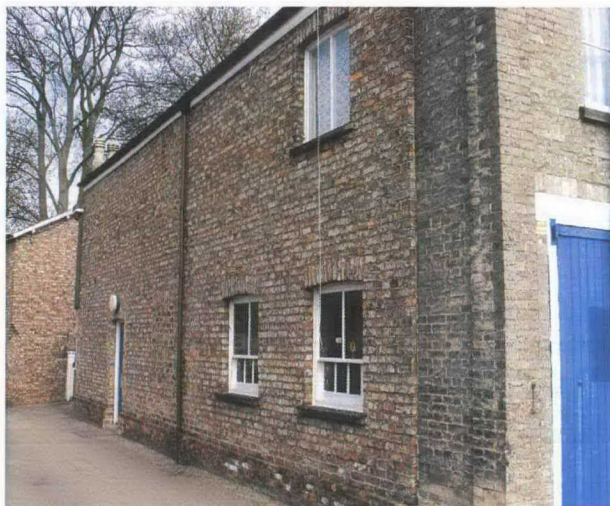
Plate 18 Refacing on Coach House
