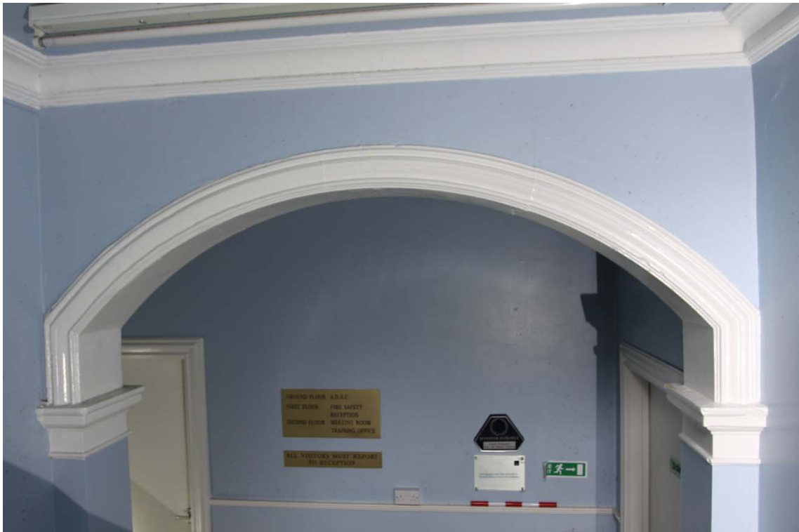
Plate 6: Room 5, archway to ground floor hall
