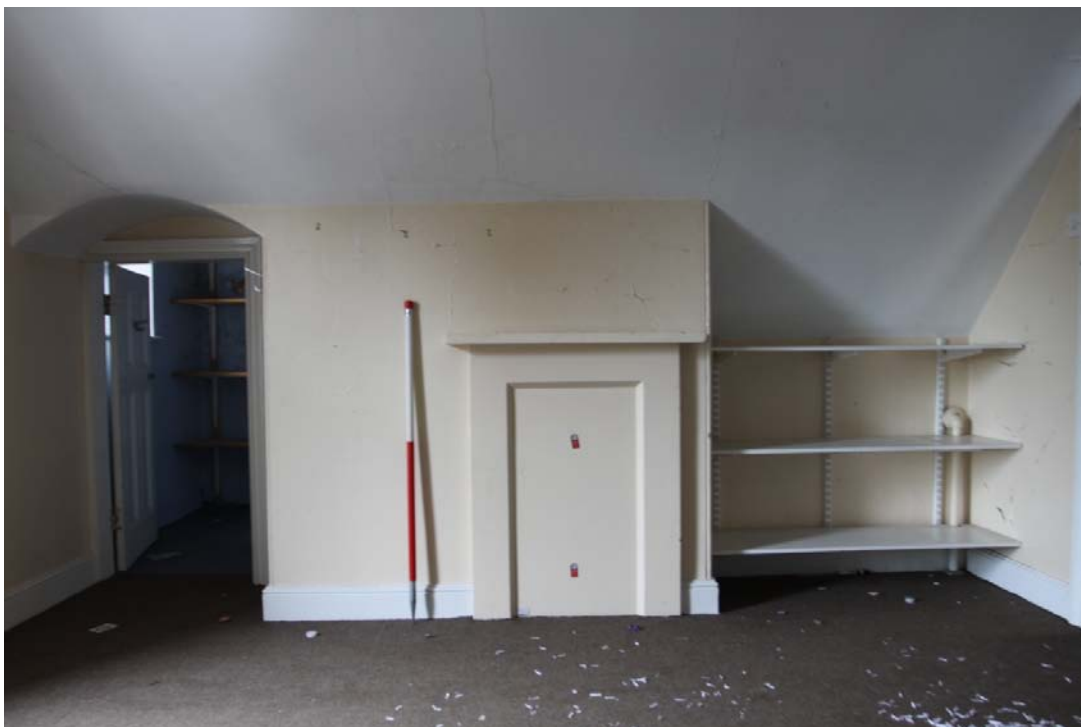
Plate 12: Room 16, south wall
