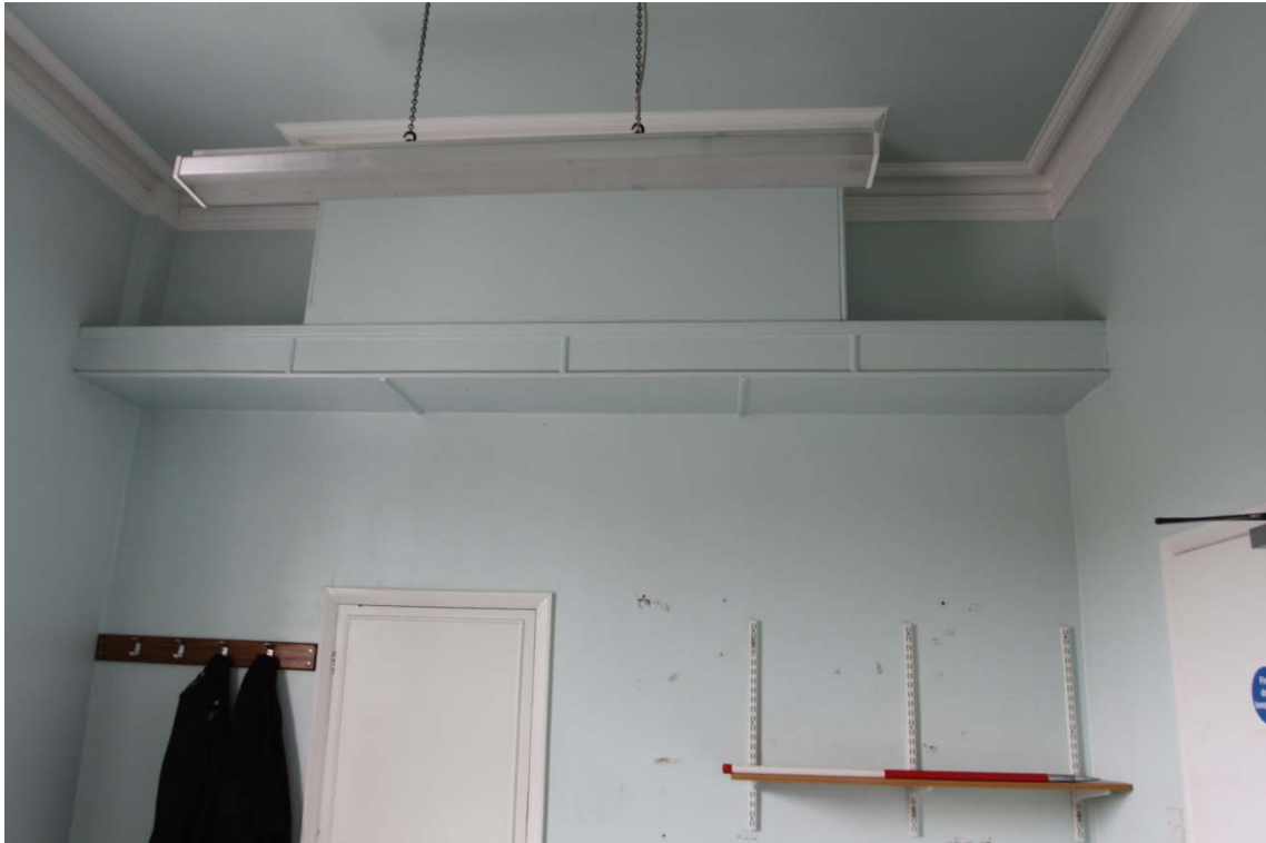
Plate 11: Room 10 former chimneystack north wall
