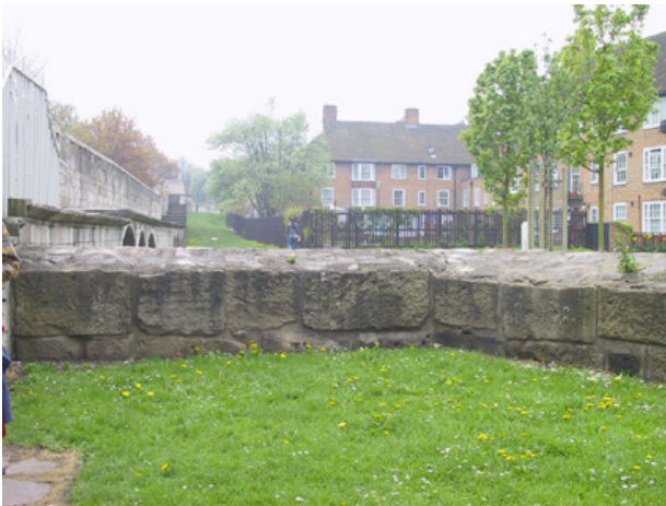
The low wall on the west side of the Red Tower, made from re-used stone blocks
