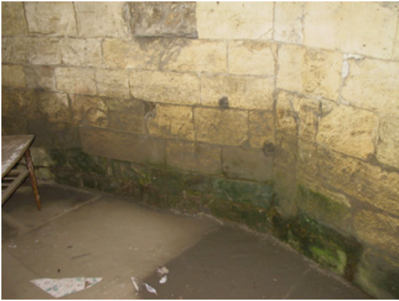
Frequent flooding and the tower's position has resulted in damp in the ground floor stonework
