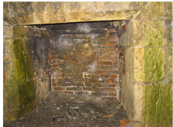
Brick backed fireplace
