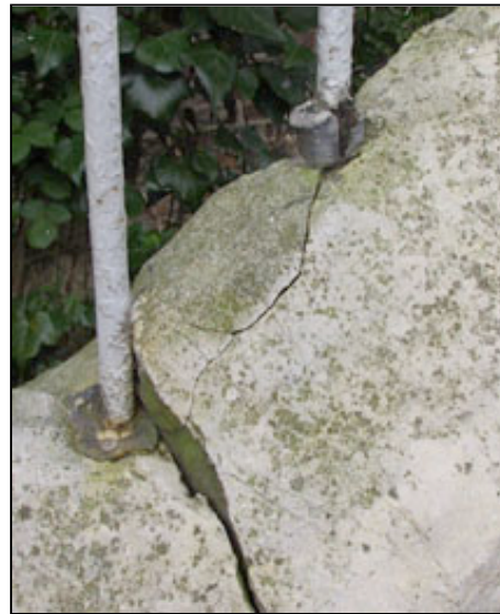
The damage that can be caused from railings can be seen here where the railings have been removed and in the picture to the right where railings are still in place near Micklegate Bar
