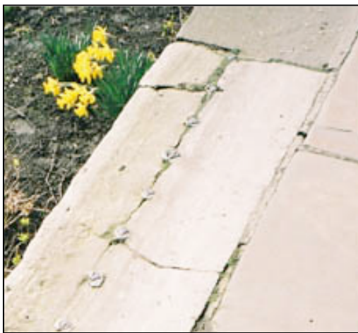
The damage that can be caused from railings can be seen here where the railings have been removed and in the picture to the right where railings are still in place near Micklegate Bar
