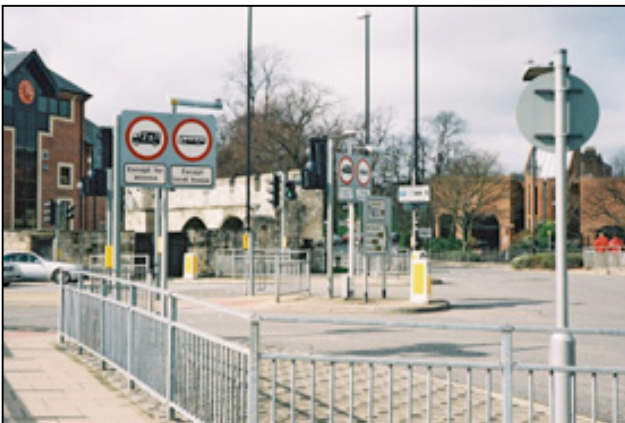
The street clutter at Layerthorpe Bridge affects views of and views from the City Walls
