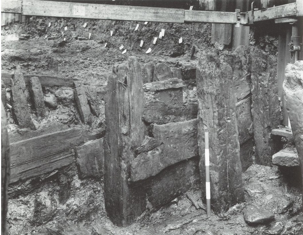
Plate 7 The walling of Building 5, scale unit 0.1m
