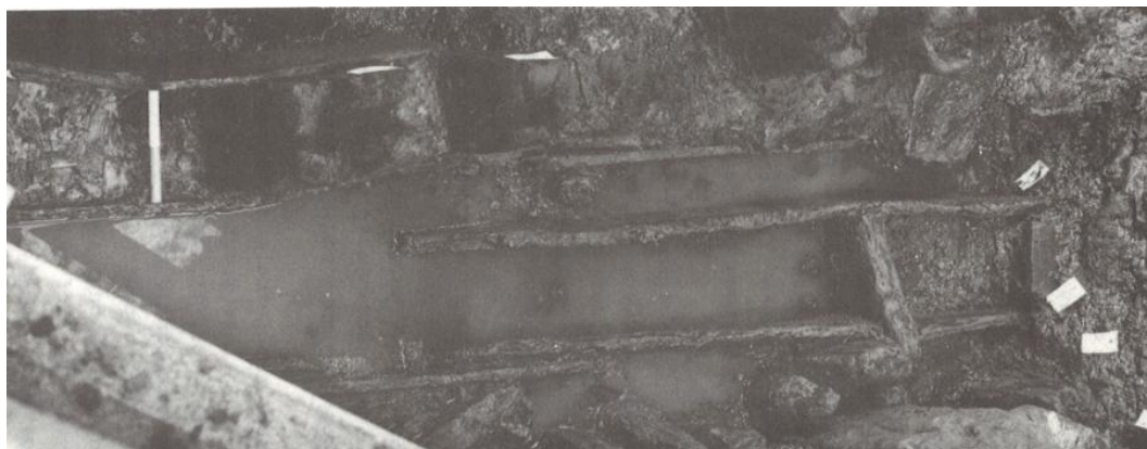
Plate 5 The timber lined drain, scale unit 0.1m
