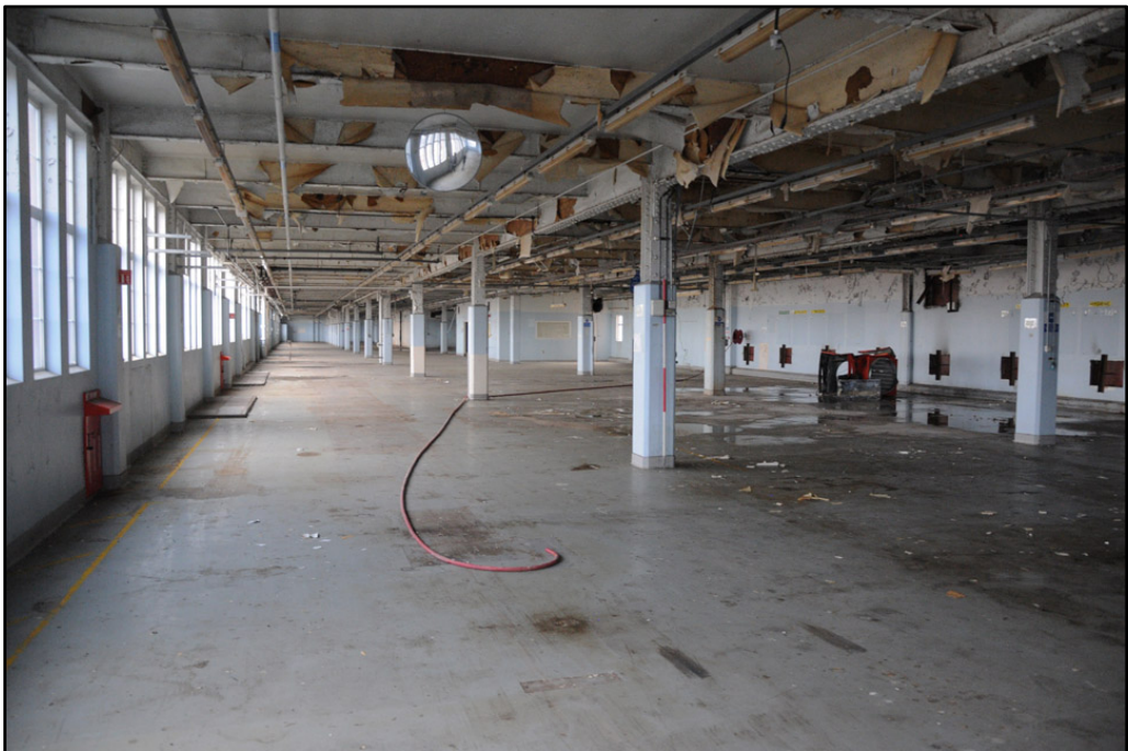
General view of sixth floor of Cream Block, looking south (2m scale)
