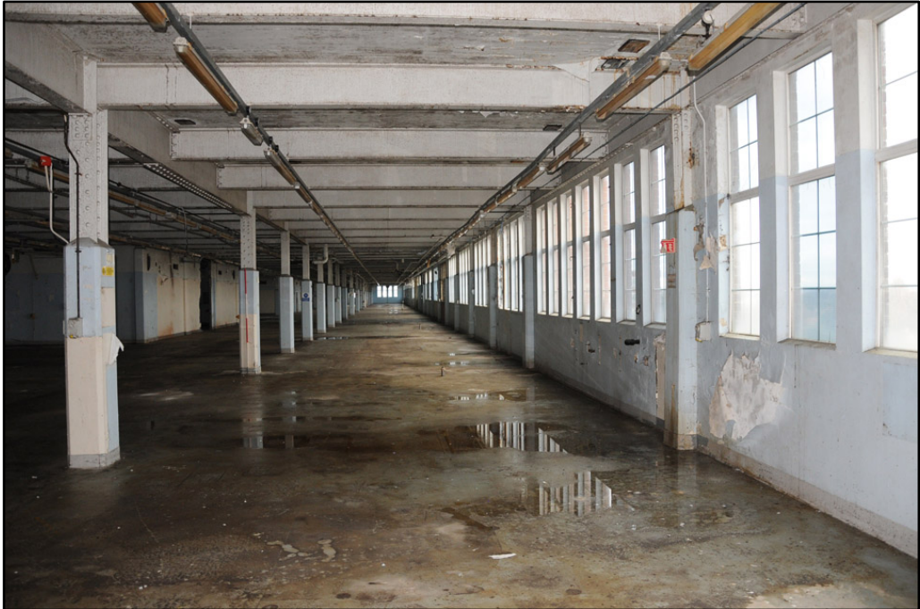
General view of sixth floor of Cream Block, looking north (2m scale))
