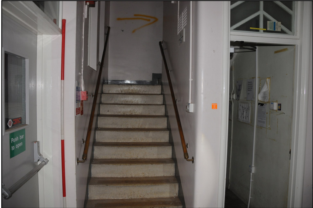
View of staircase at north end of three-storey section of Cream Block; note timber handrails (2m scale)
