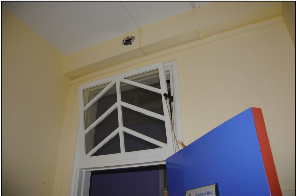
Detail of decorative fanlight in 1936 three-storey section of the Cream Block
