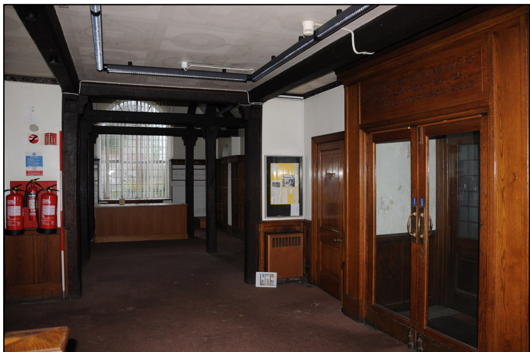
General view of entrance foyer in Joseph Rowntree Library, looking north (2m scale)
