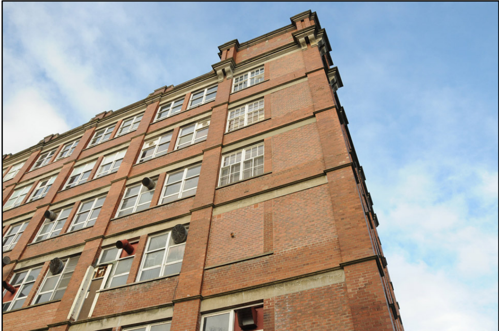
View looking up of southeast corner of Almond Block; note original windows with small lights
