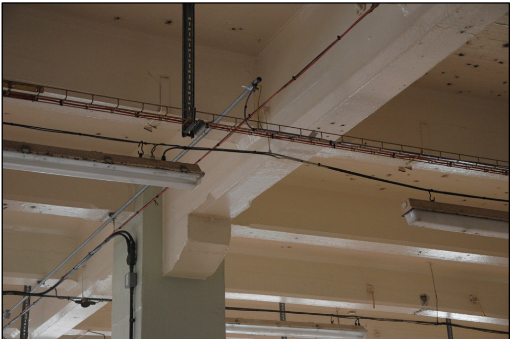
Detail of cast concrete decoration on third floor of Almond Block
