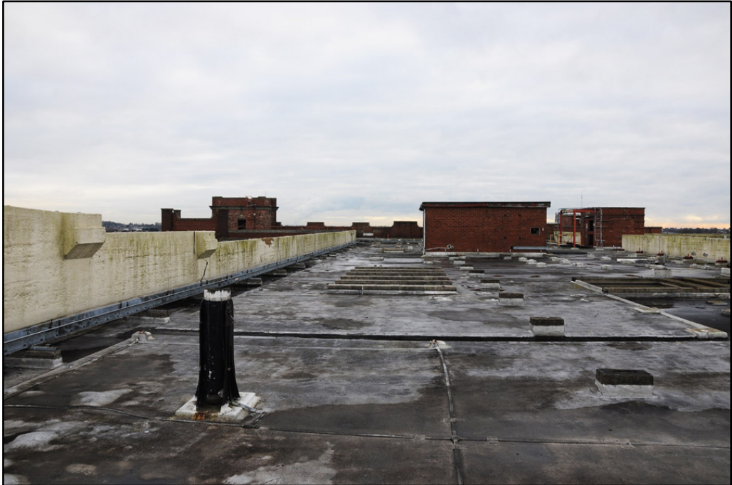
View looking south across flat roof of Cream Block; note sawn off base to flagpole
