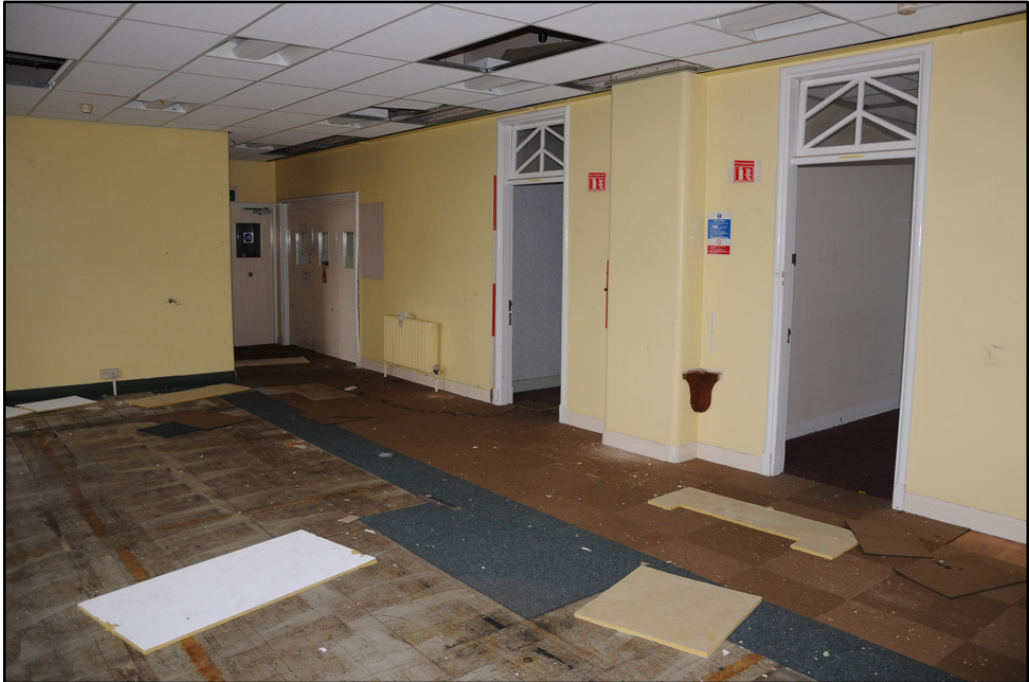
Detail of first floor rooms in 1936 three-storey section of the Cream Block (2m scale)
