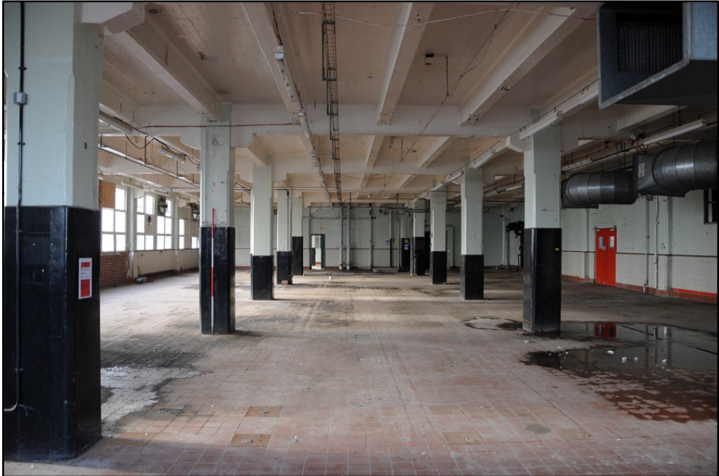
General view of third floor of Almond Block; note exposed concrete superstructure (2m scale)
