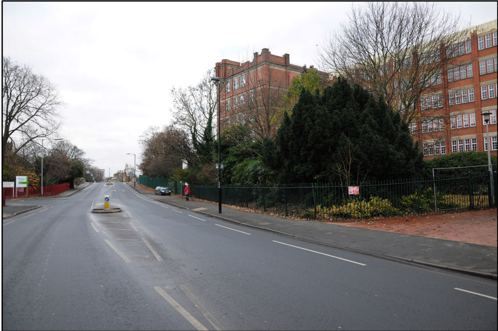
General view looking south along Haxby Road, note extent of railings and overgrown shrubbery
