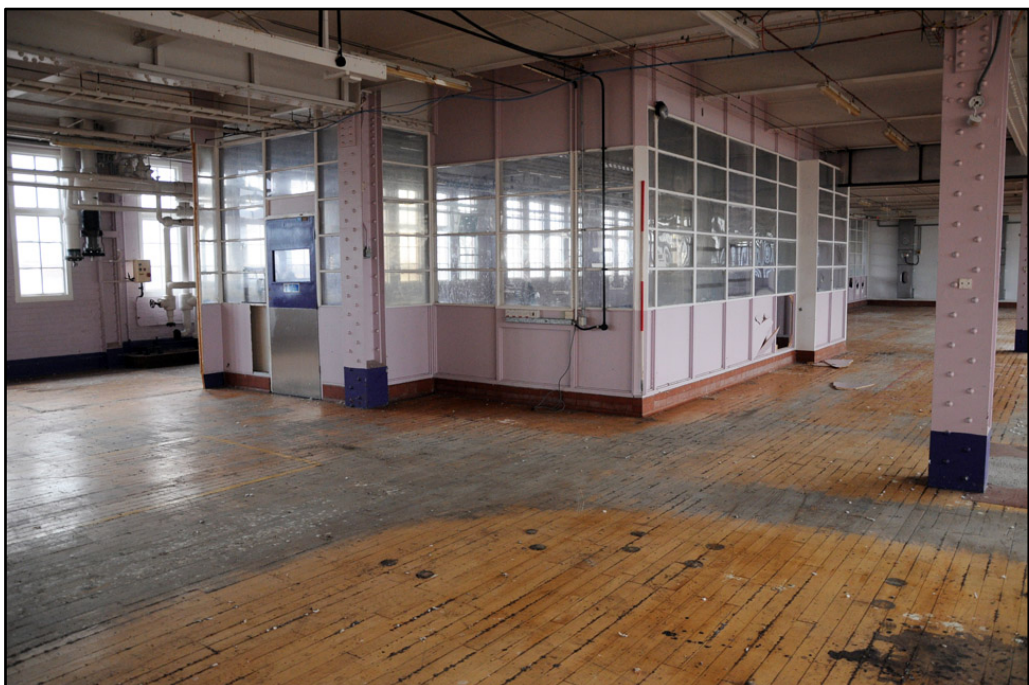
Detail of inserted office within fifth floor of Cream Block; note ware pattern in floor (2m scale)
