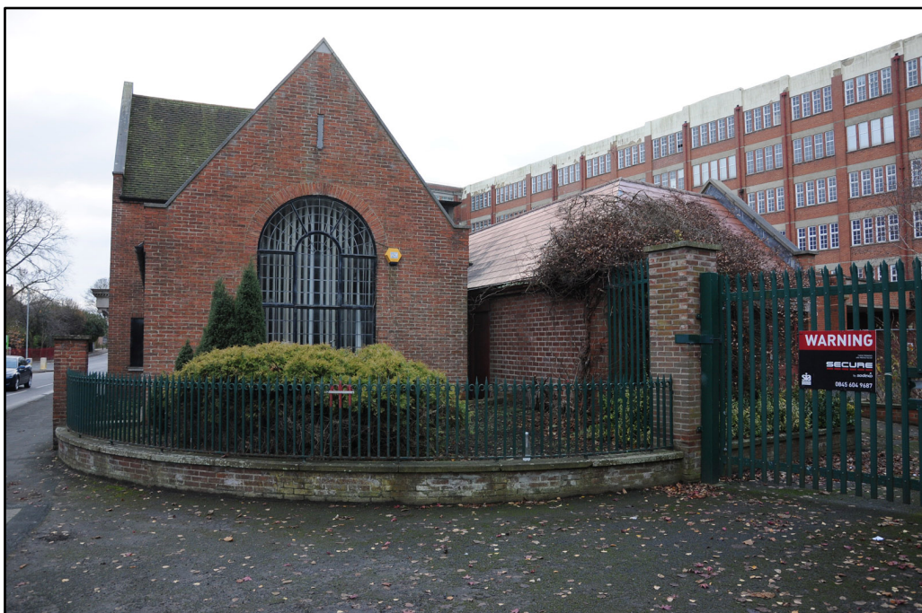
General view of north gable of Joseph Rowntree library looking south; note modern security gates
