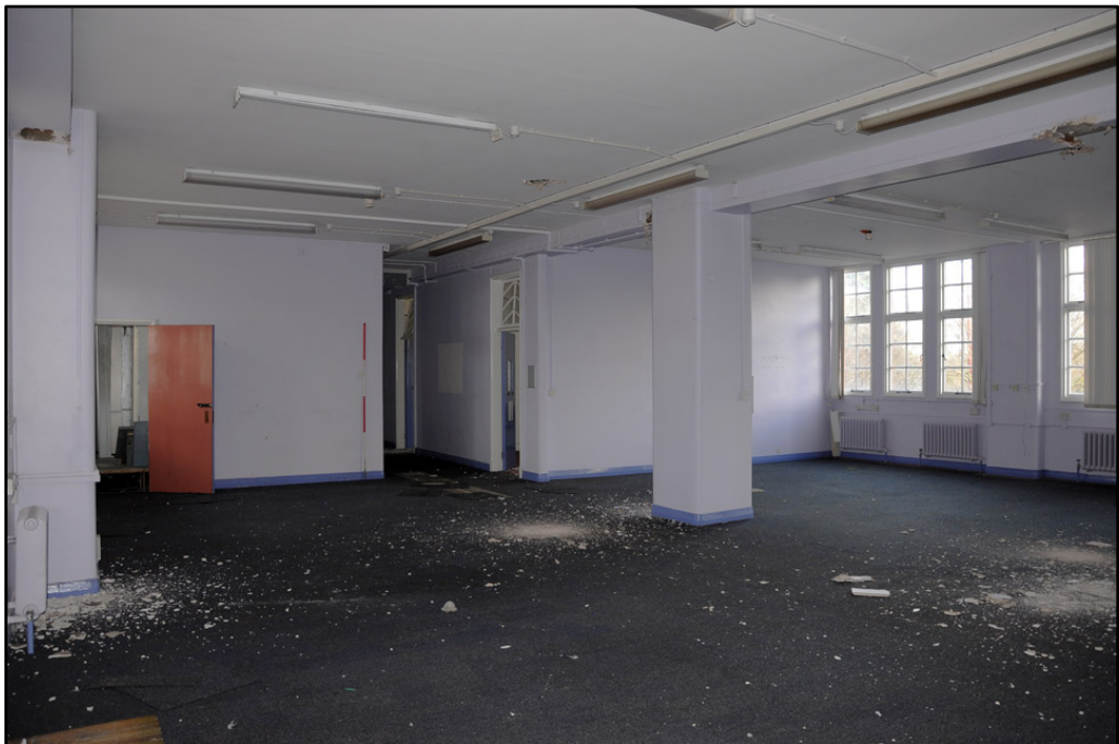
Detail of second floor rooms in 1936 three-storey section of the Cream Block (2m scale)
