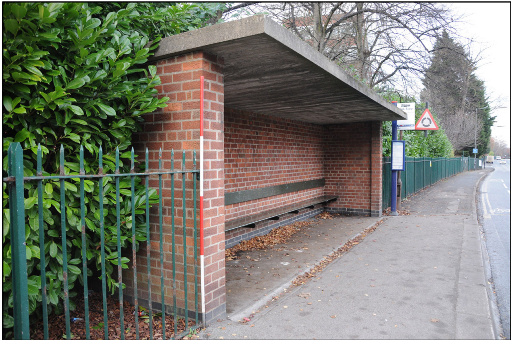
Detail of bus stop on west side of Haxby Road, looking north
