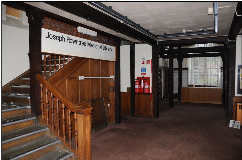
General view of entrance foyer and staircase in Joseph Rowntree Library, looking north (2m scale)
