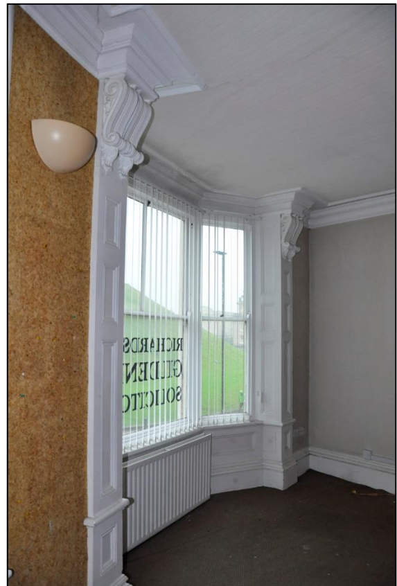
Figure 13: Victorian window surround with decorative console brackets to first floor window
