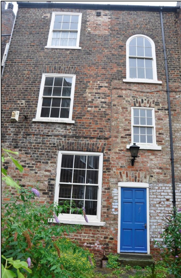
Figure 14: Rear elevation; note areas of infill and rebuilding and a number of modern window units
