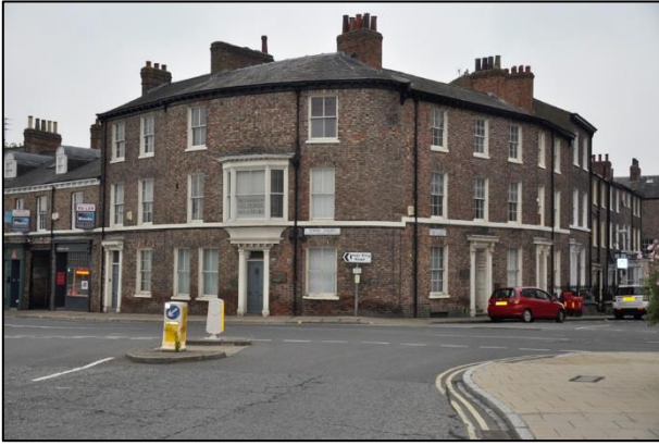
Figure 10: Frontage to application site
