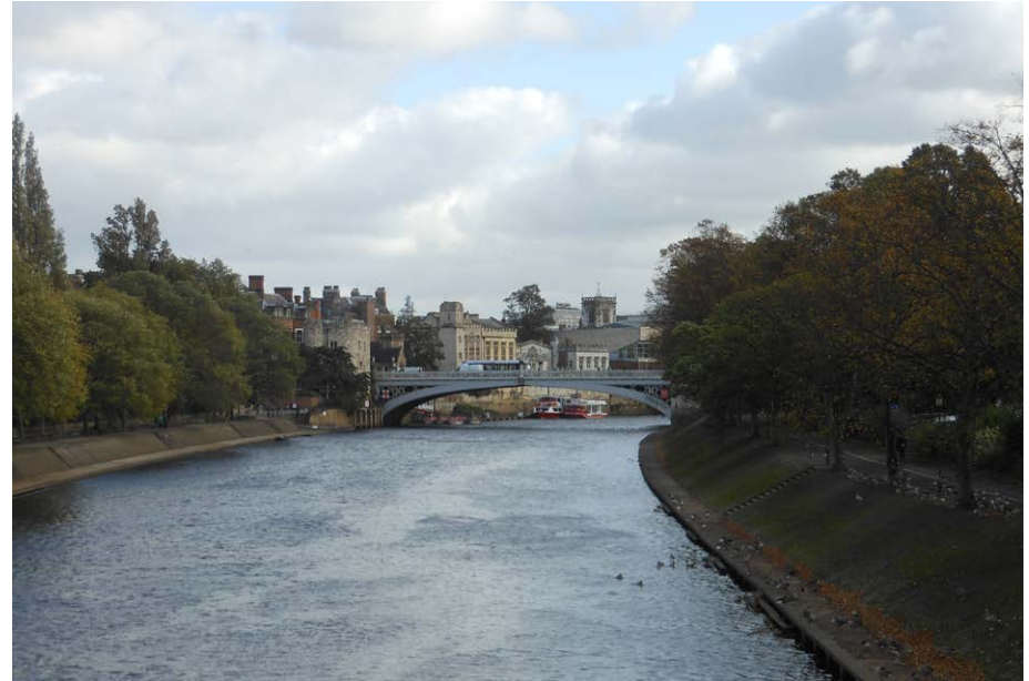
Fig. 22: View from the footway on Scarborough Bridge towards Lendal Bridge.
