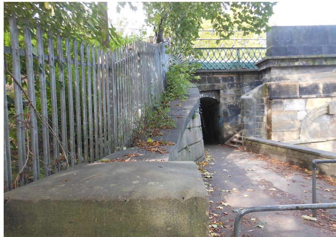
Fig. 11: South-east wing wall.
