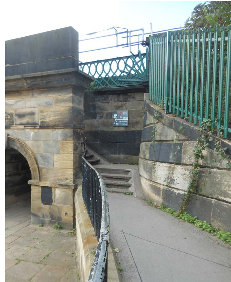
Fig. 9: The east side of the northern abutment.
