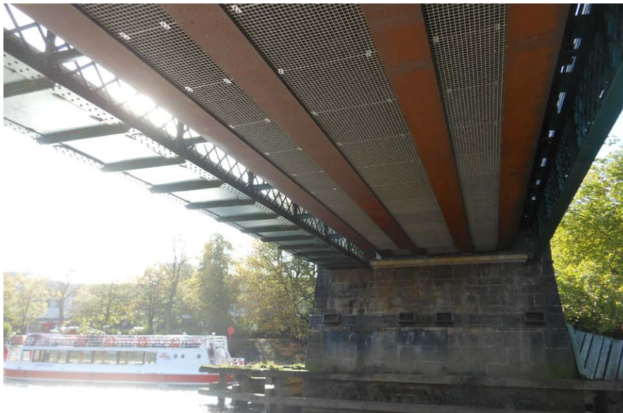
Fig. 13: Underside of the bridge showing the new steel deck.
