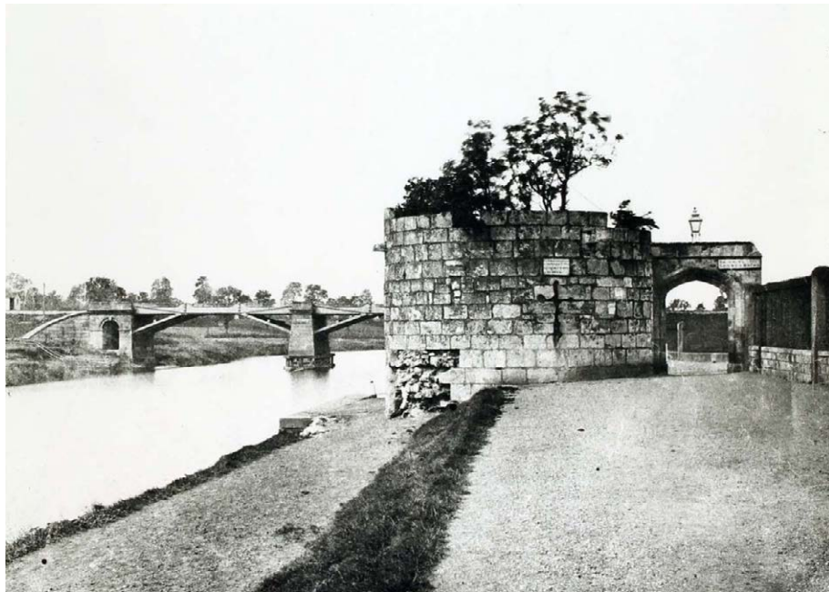
Fig. 5: View of the bridge from the east, c.1850s–60s. Note the bracing under the deck of the bridge which was added after 1847.
