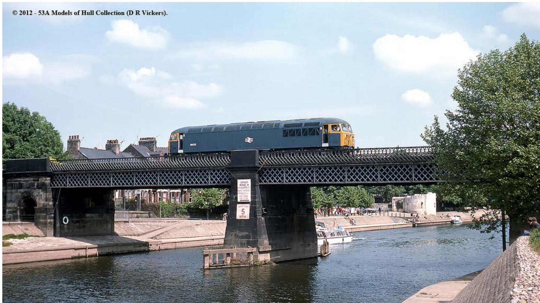
Fig. 12: View of the west side of Scarborough Bridge, 9 June 1977.
