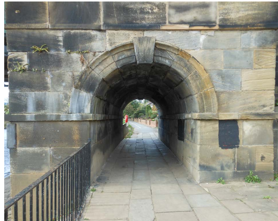
Fig. 4: Detail of stonework on the northern abutment.
