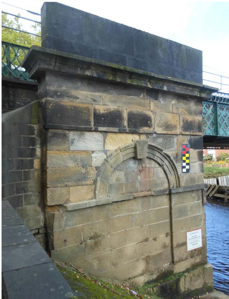
Fig. 10: The east side of the southern abutment, showing the infilled archway.
