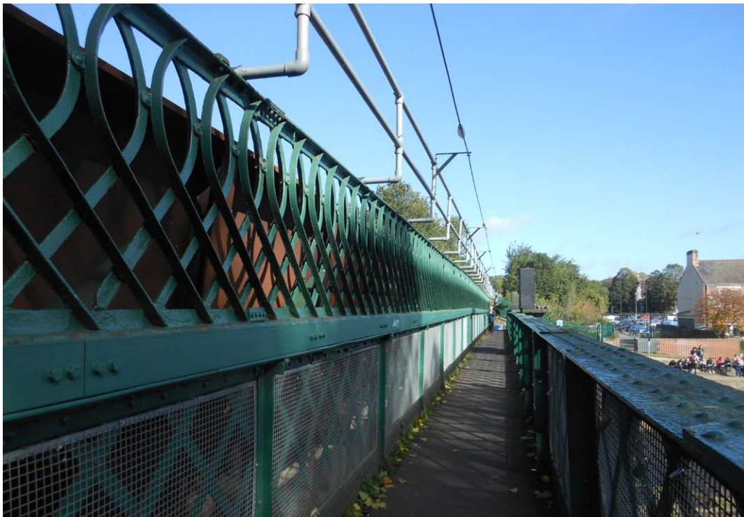
Fig. 8: The footway on the east side of the bridge, looking north.
