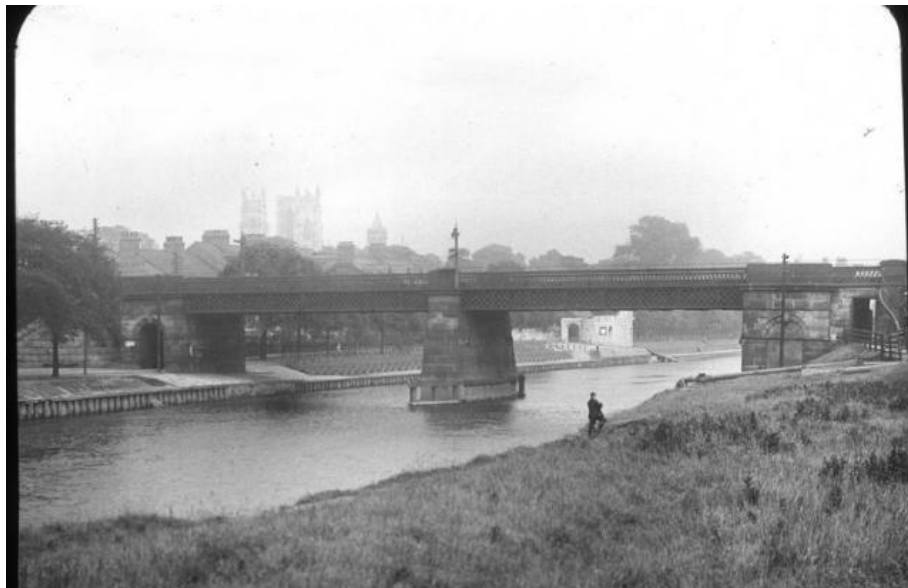
Fig. 18: West side of the bridge, c.1912.
