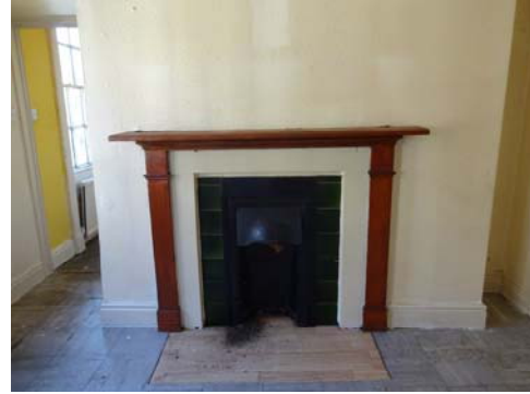
12 Castlegate 1 st Floor Fireplace
