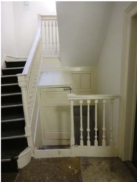
Staircase at No. 14 Castlegate.
