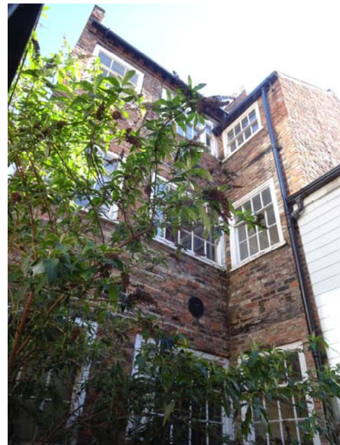
Windows to rear elevation of No. 12
