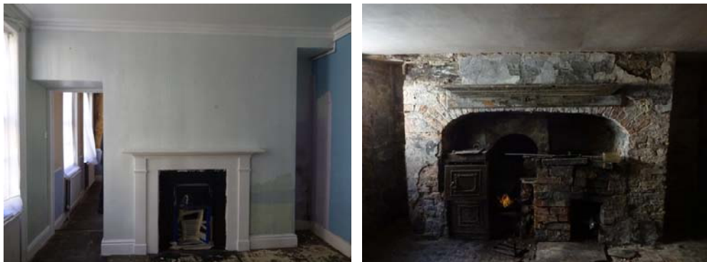
12 Castlegate Ground Floor Fireplace and Basement Range
