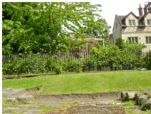
Plate 8 – Physical Barriers to Access
