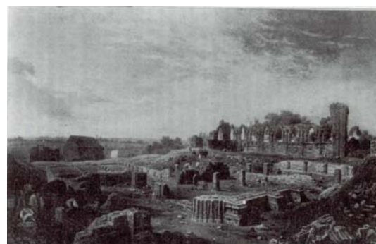
Plate 10 – Excavated Remains of the Abbey Church
