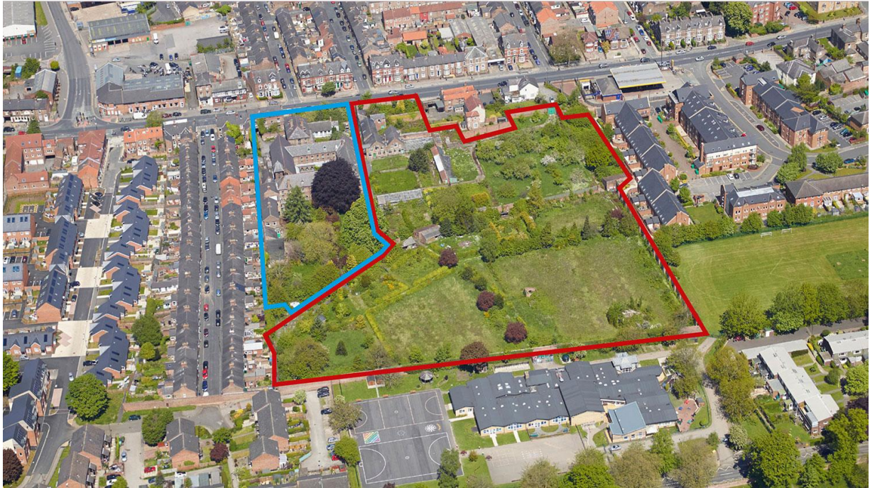
Figure 2: Physical map of the site with the excavation and development area bound in red and the existing buildings of St Joseph's and associated convent graveyard bound in blue.
