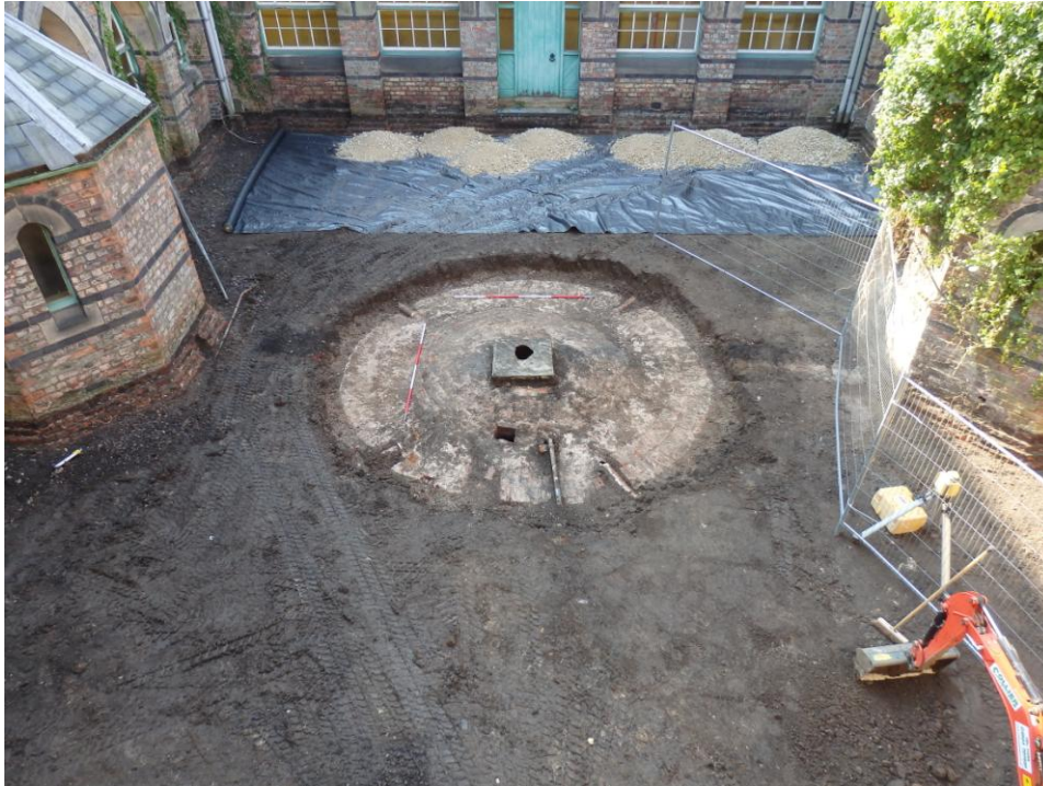
Plate 35: Domed brick well/cistern located in the courtyard/cloister [368].
