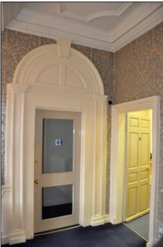
Figure 23: Doorcase in east wall of landing with modern door and 18 th century eight panelled door to former saloon
