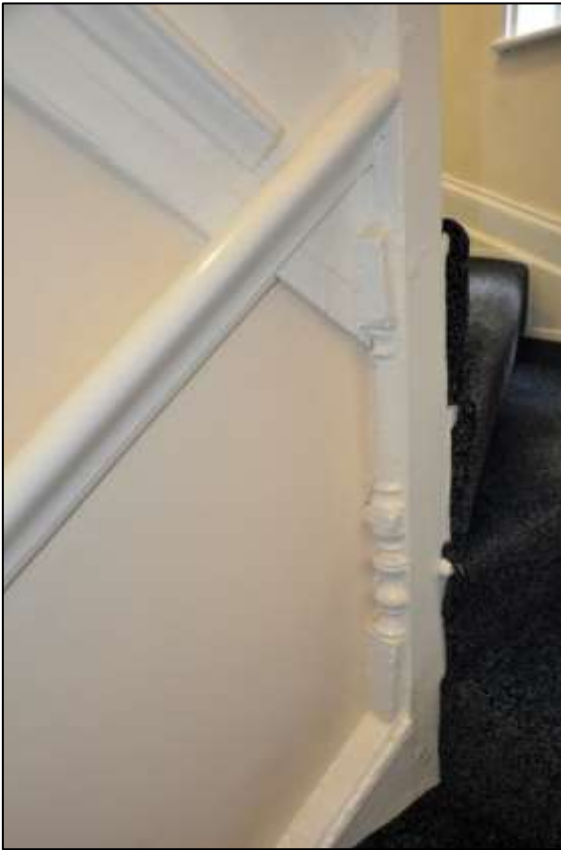
Figure 25: Example of surviving early 19 th century baluster to stairs to second floor
