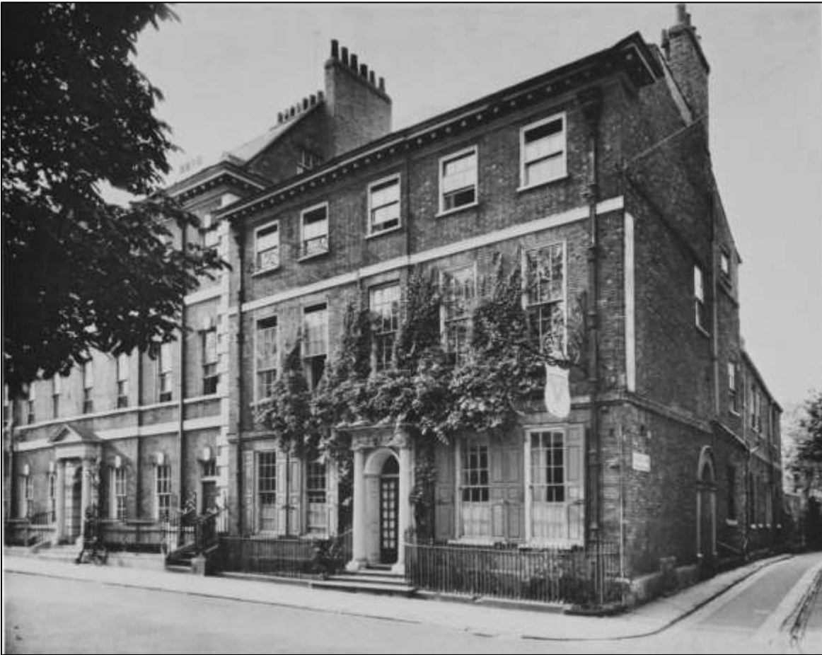
Figure 11: Bathurst House in c.1964 (© RCHME)
