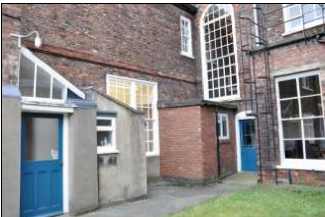
Figure 18: Mid-late 20 th century single storey, single bay extensions to the rear of the north elevation of the house
