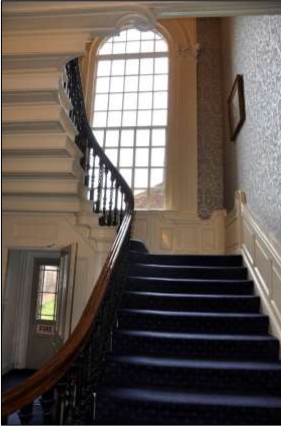
Figure 22: Staircase and window with detail of balusters (right)
