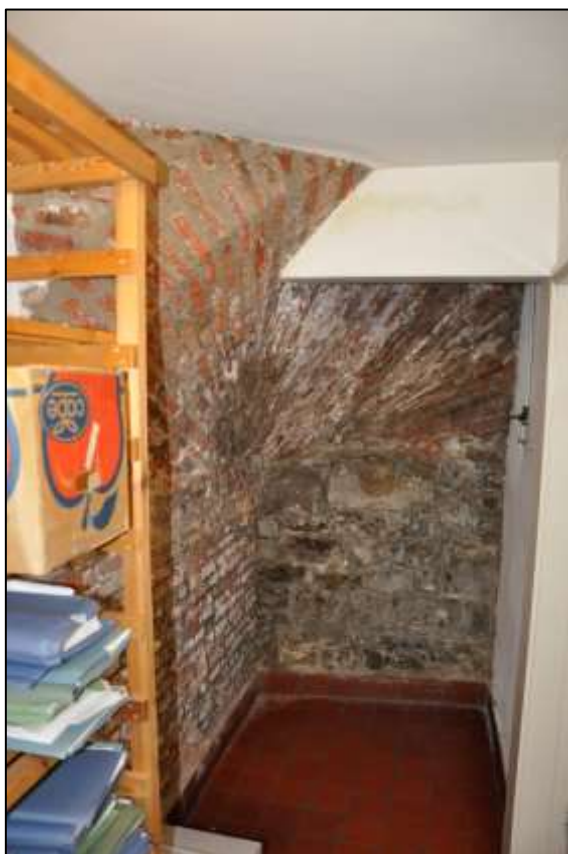
Figure 20: Medieval wall supporting later brick vaulting in basement
