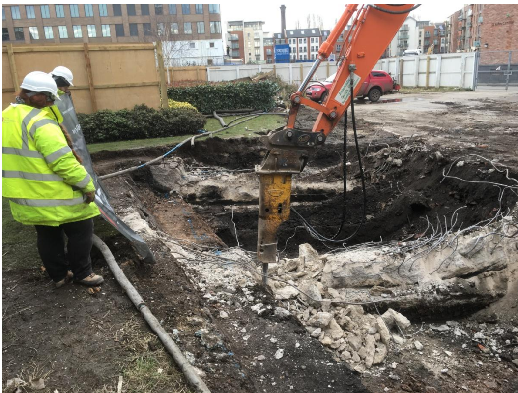
Plate 11 Machine excavation of concrete footings (Group 36002)
