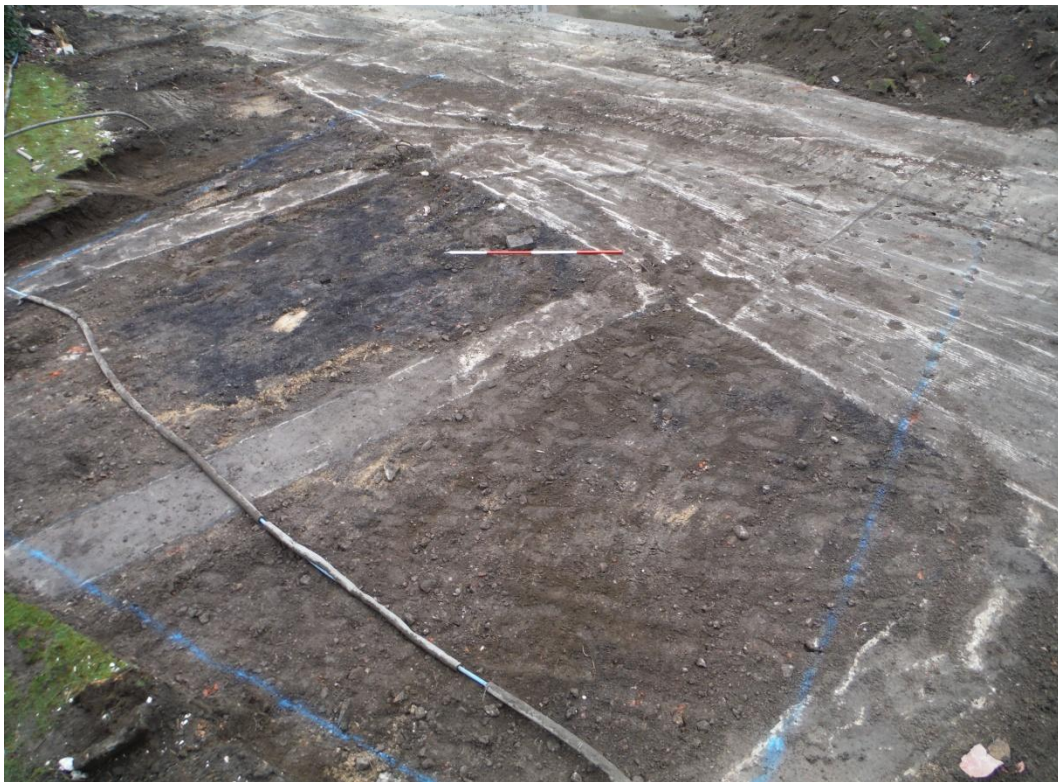
Plate 10 South-east facing, pre-excitation view of 20th century concrete footings (Group 36002, 2.00m scale)
