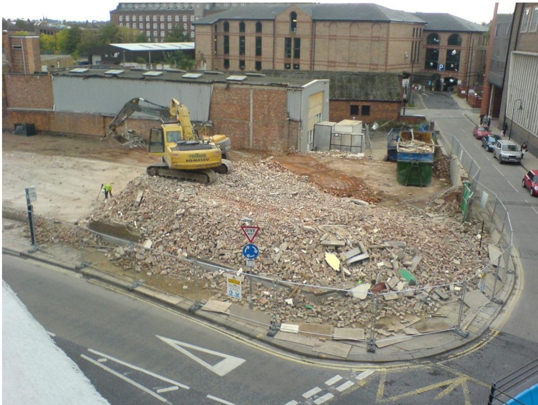
Plate 19 Warehouses on Block G during demolition in 2006 (courtesy of David Dodwell)
