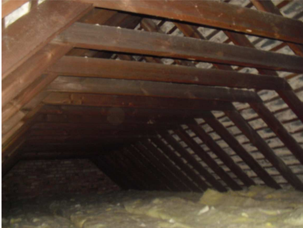
Fig 10: College 1 studies: 1956 roof and brickwork of gable
