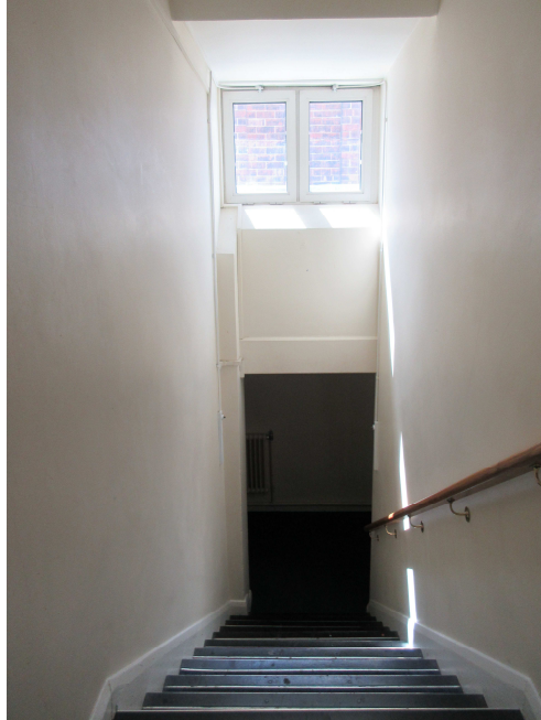
Fig 5: Existing staircase to 2 nd floor level.
