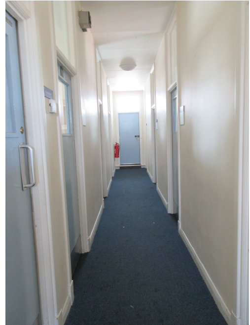
Fig 6: Existing 2 nd floor corridor looking towards timber fire door.
