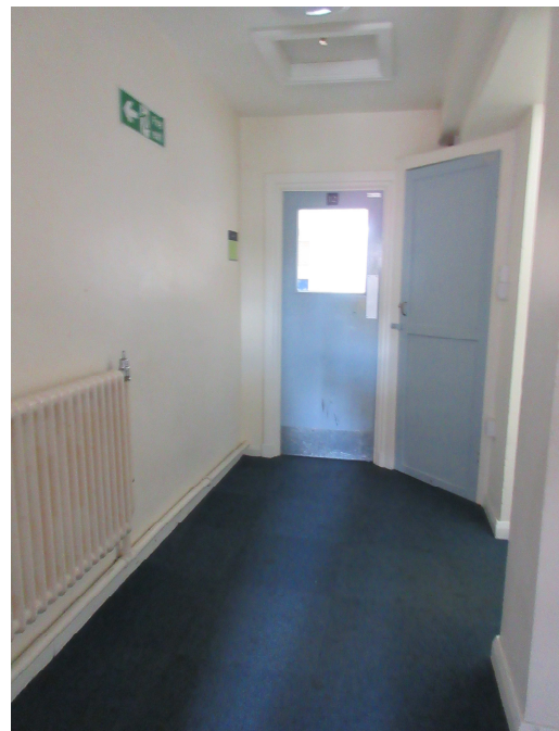
Fig 4: First floor study. Stairway to right hand side.
