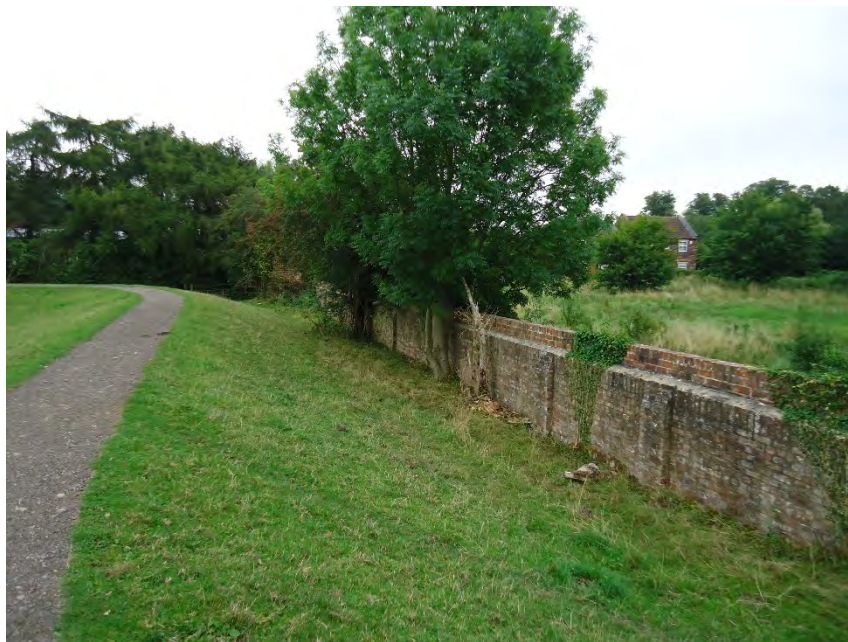
Plate 9: Looking north-east along the extant former asylum boundary wall
