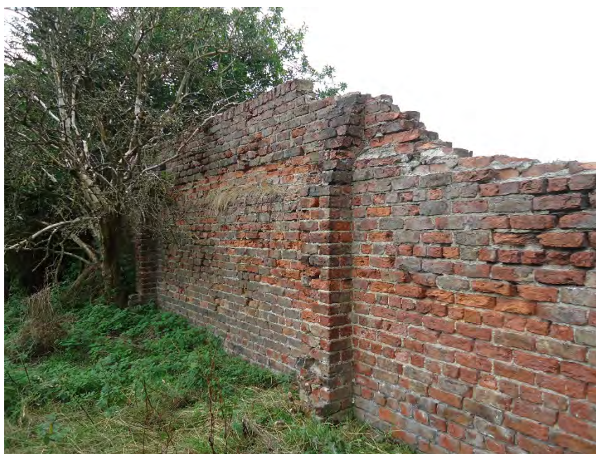
Plate 8: Looking north-west at part of the extant former asylum boundary wall
