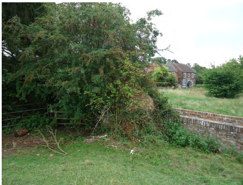
Plate 10: Looking north-east along the extant former asylum boundary wall/structure
