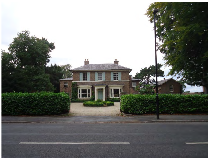
Plate 3: Looking south-west towards 25 Shipton Road (NHLE 1256626)
