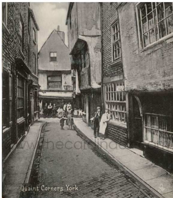
No.1 Little Shambles (L) seen far left in 1929 with the second floor propped © YAYAS; and (R) seen far right in the late C19/early C20 showing considerable lean in the front elevation © www.thecardindex.com.
