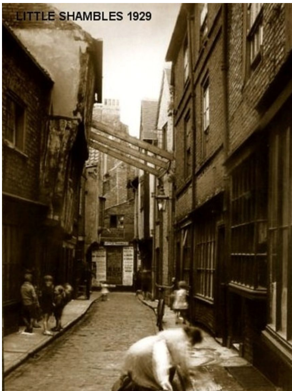
No.1 Little Shambles (L) seen far left in 1929 with the second floor propped © YAYAS; and (R) seen far right in the late C19/early C20 showing considerable lean in the front elevation © www.thecardindex.com.
