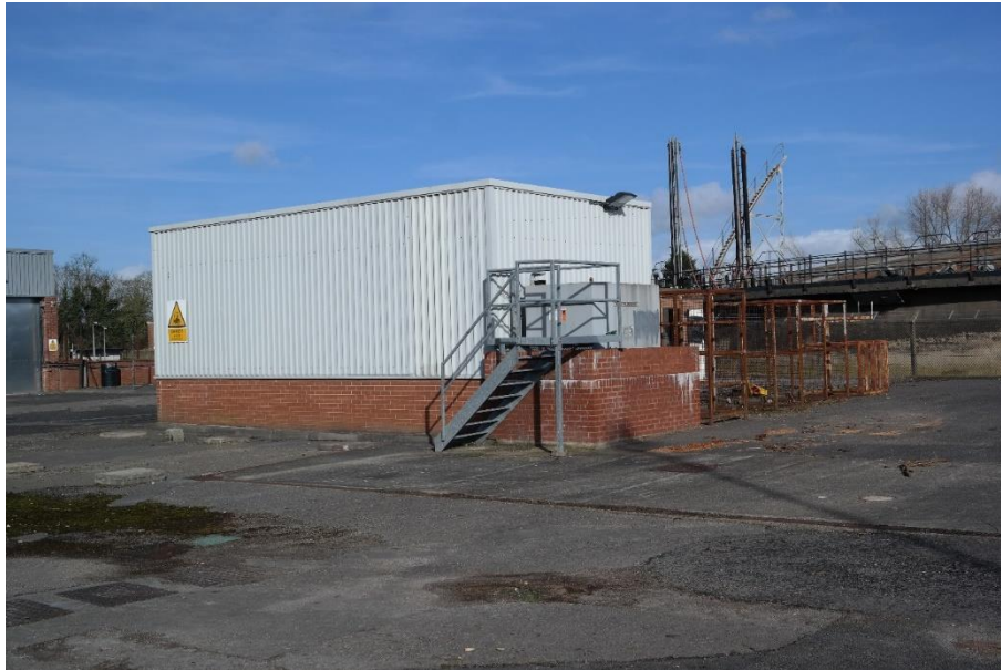
Plate 42 the metal buildings to the west of the gas storage tank facing north-east
