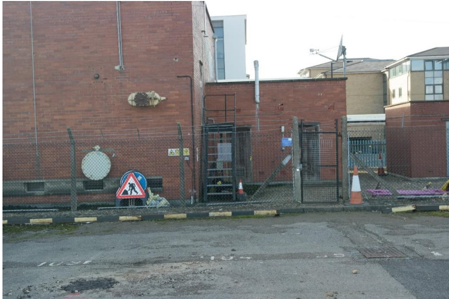
Plate 14 Zone B buildings facing west
