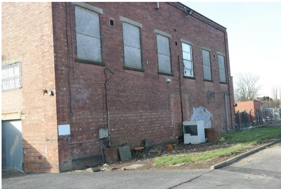
Plate 13 Zone B buildings facing north-west
