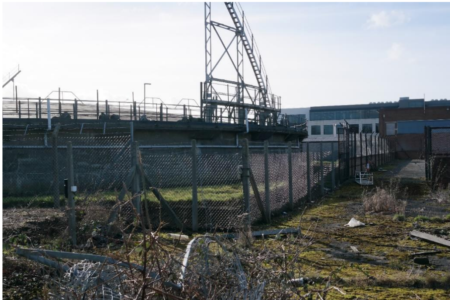
Plate 39 Zone F the gas storage tank facing south-west
