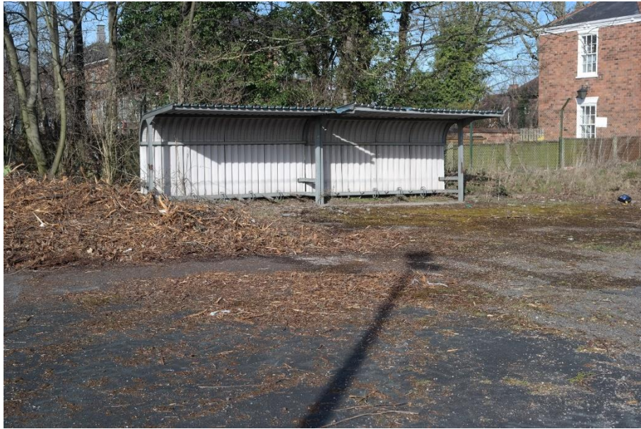
Plate 32 The bike sheds in Zone D facing north
