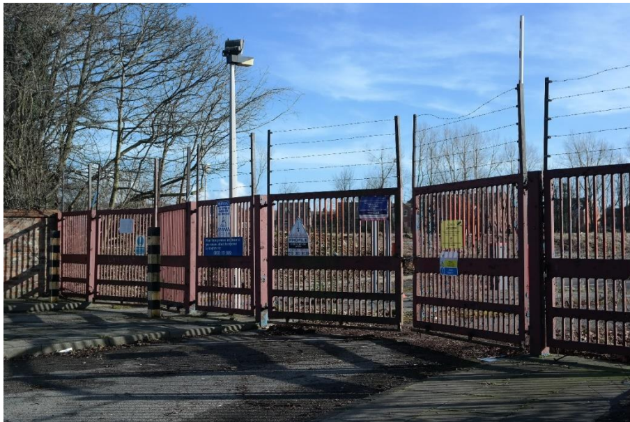
Plate 21 Zone D the metal access gates for the site facing south-east
