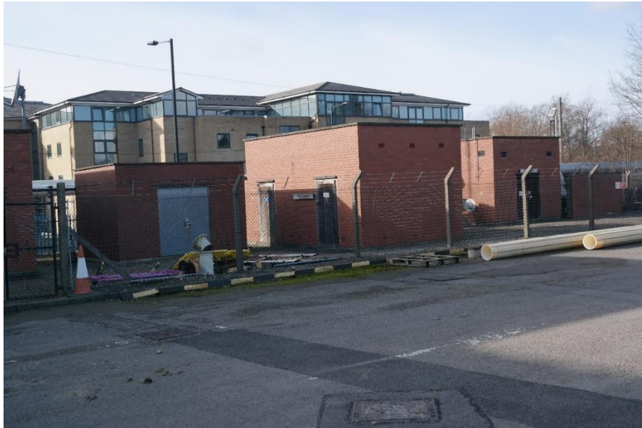
Plate 10 Zone B buildings facing west
