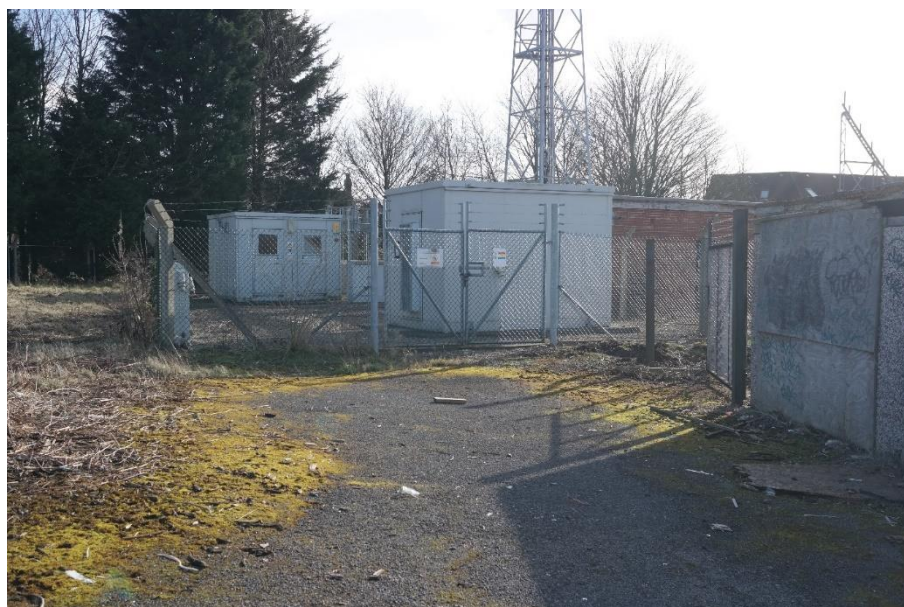
Plate 45 Small cabins to the east of the gas storage tank
