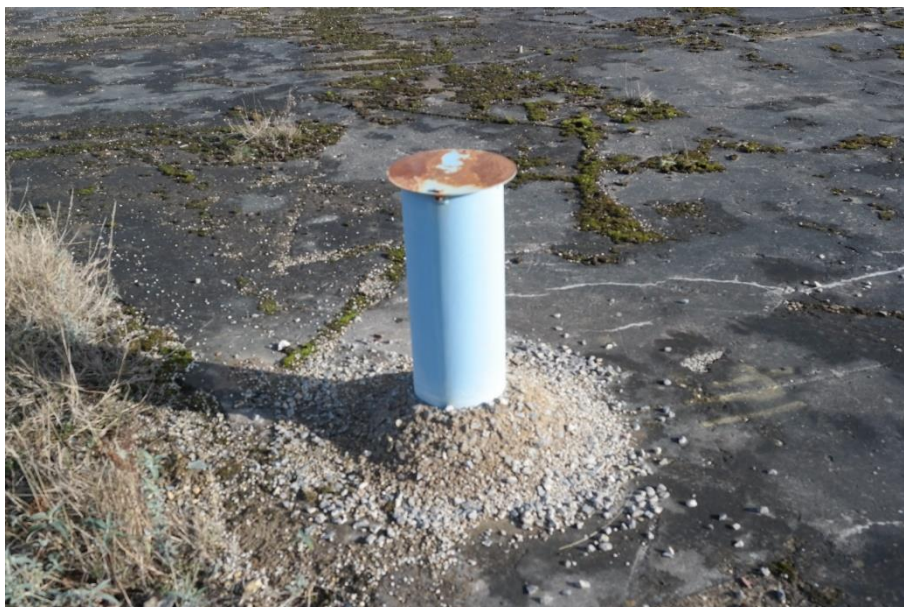
Plate 29 Metal pipes on the building plinth of Zone D facing east
