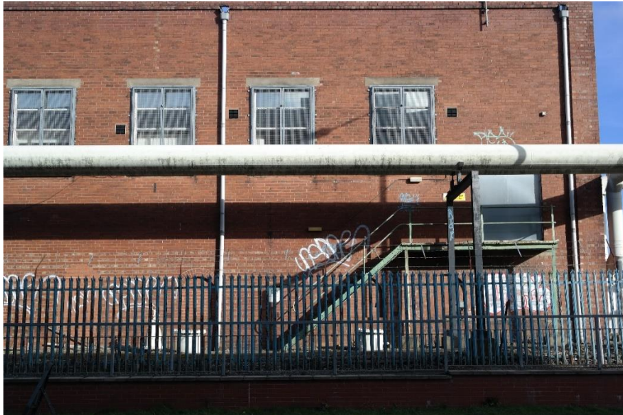
Plate 12 Zone B facing east. Graffiti on the main building and the major pipeline.
