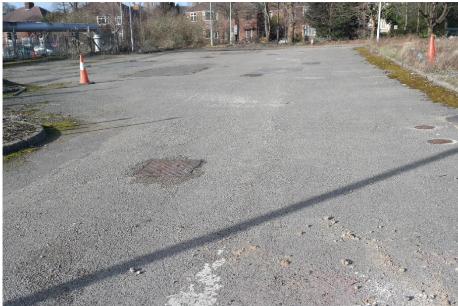
Plate 27 The westernmost road of Zone D facing north
