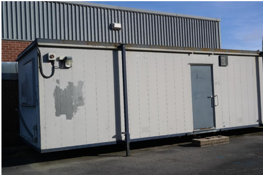
Plate 43 A portacabin to the west of the gas storage tank
