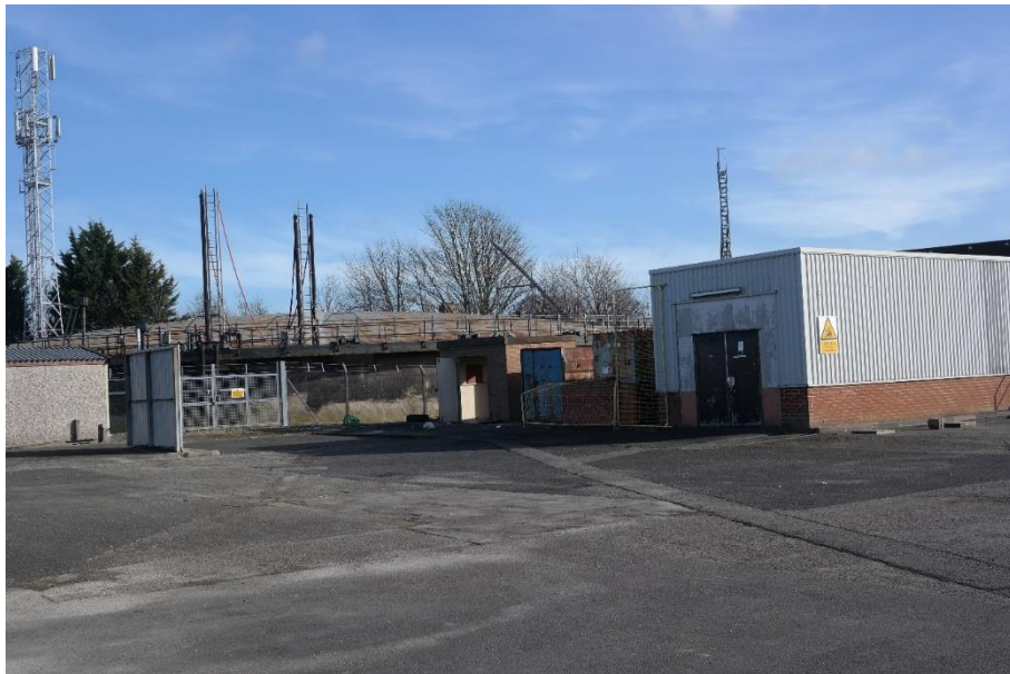
Plate 41 the metal buildings to the west of the gas storage tank facing east
