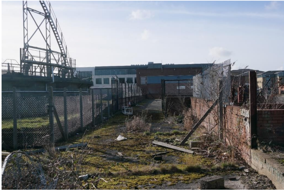
Plate 40 The area to the immediate north of the gas storage tank facing west
