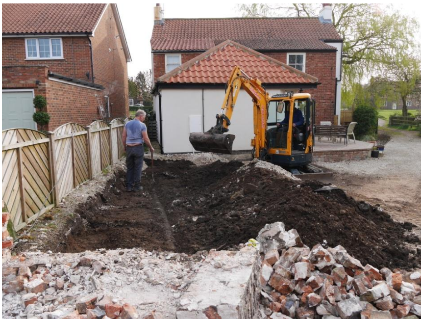
Figure 2: Image showing the excavation of the foundation for the new extension. Looking east
