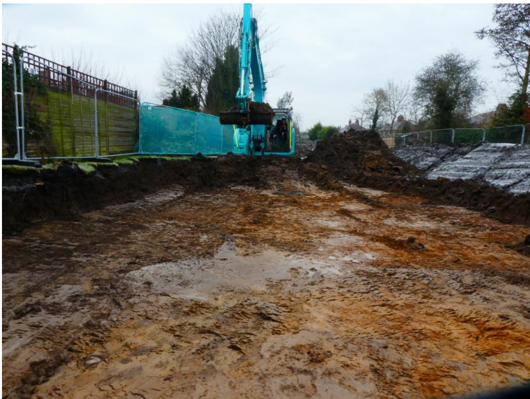
Plate 4: Stripping the site. Facing Southeast.
