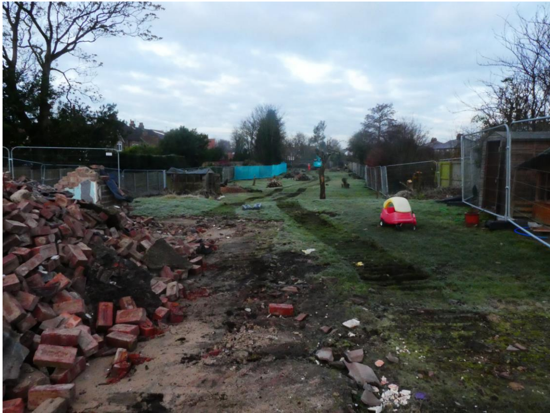
Plate 1: General view of the site. Facing North-West.
