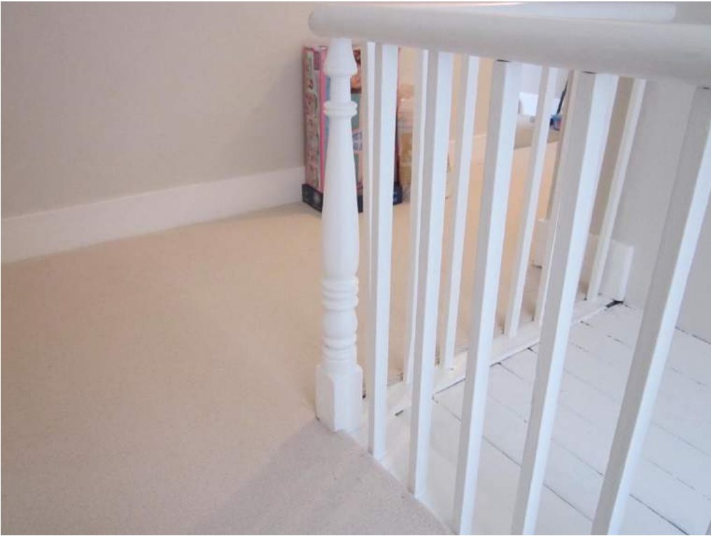
Fig 6: Attic floor: head of Phase I service stair
