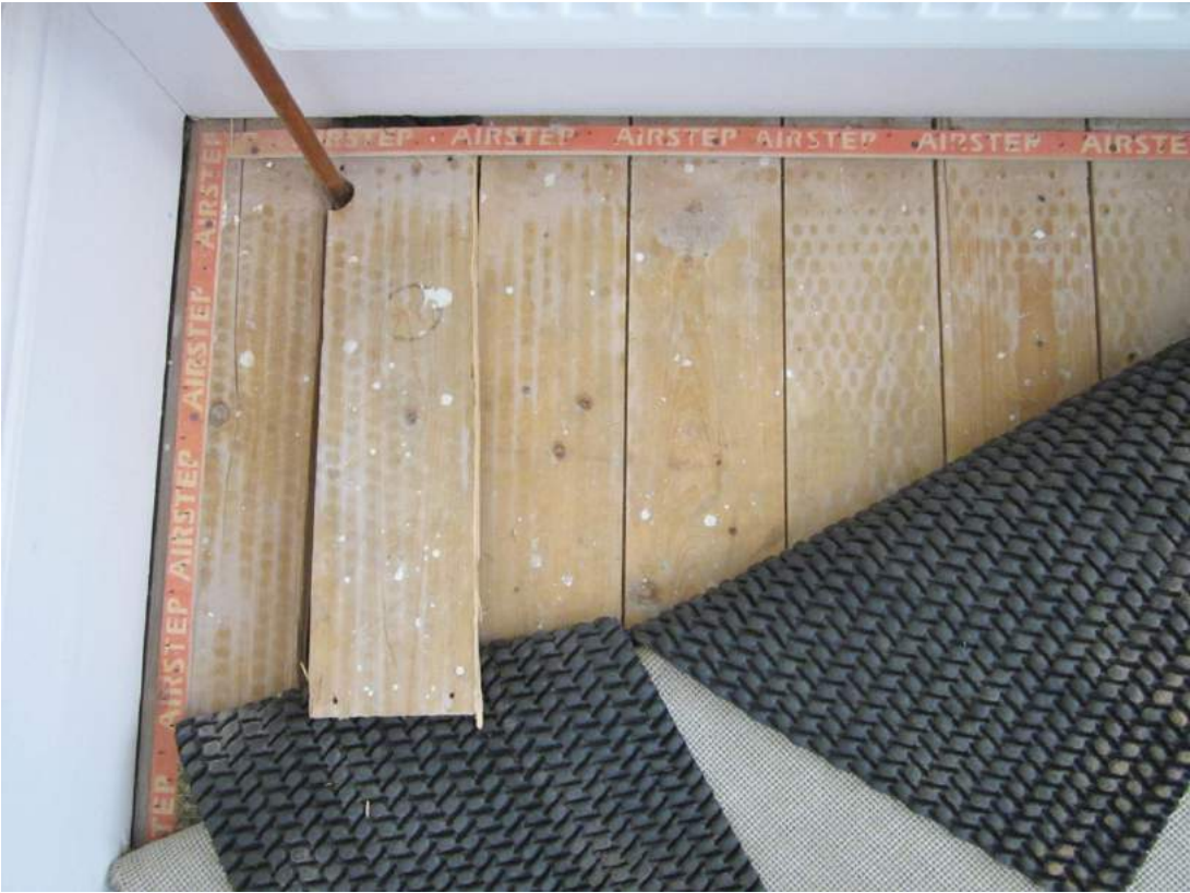
Fig 18 Inserted floor of c.1980 in former Phase I stair hall
