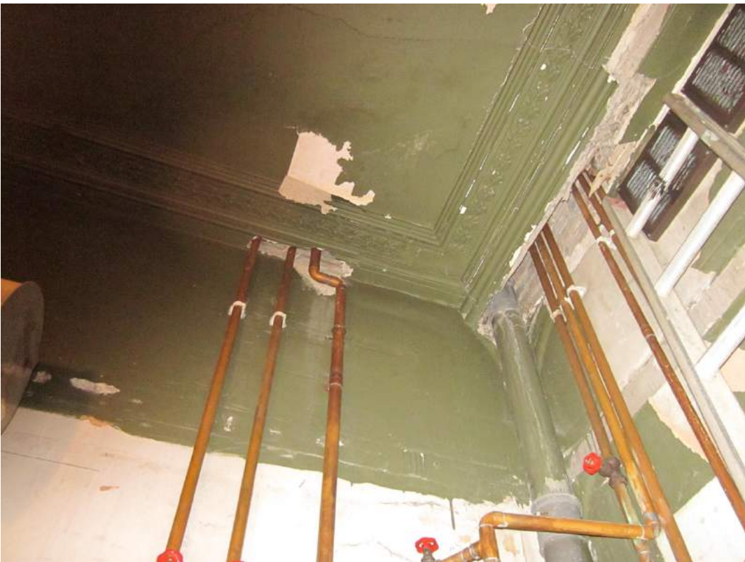
Fig 13 Fragment of Phase I moulded plaster ceiling cornice to NW corner of lost Saloon
