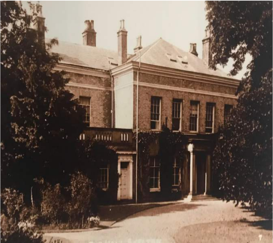
Fig 24 The Hall in c.1920
