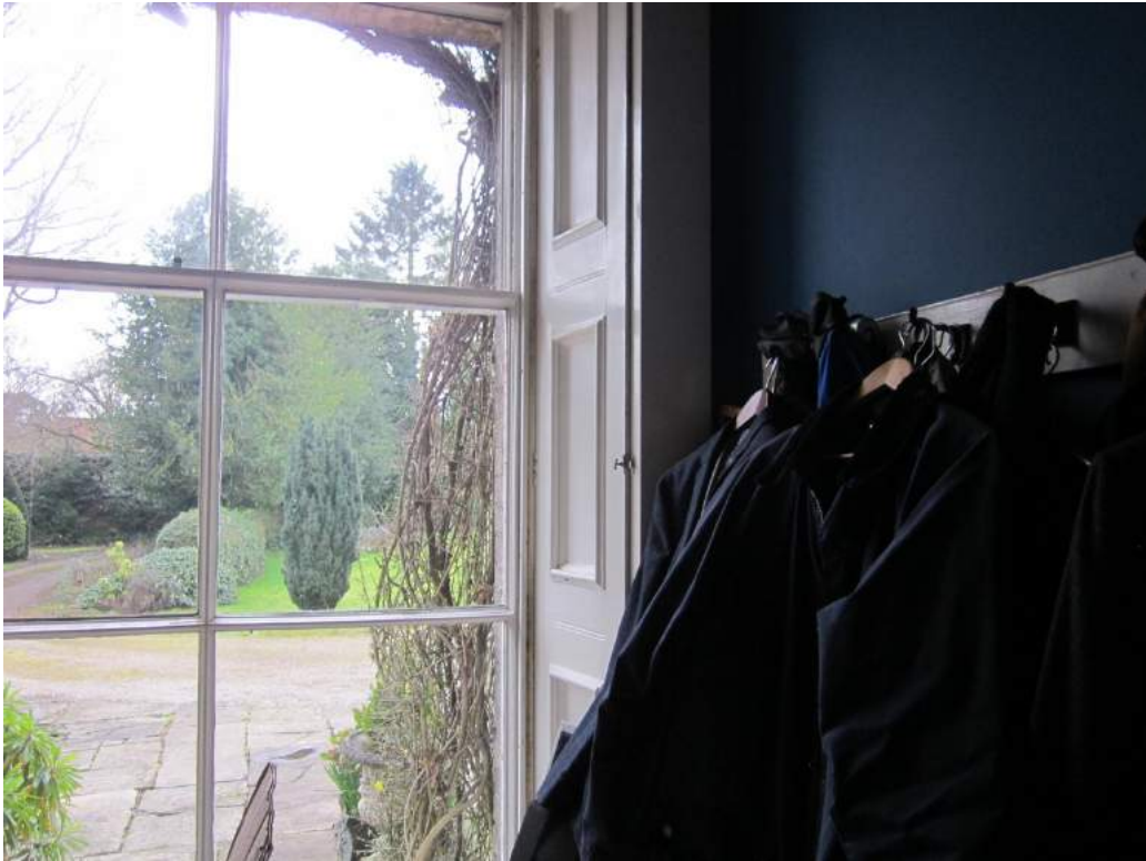
Fig 10: Cloakroom: detail of Phase I beaded folding panelled shutters
