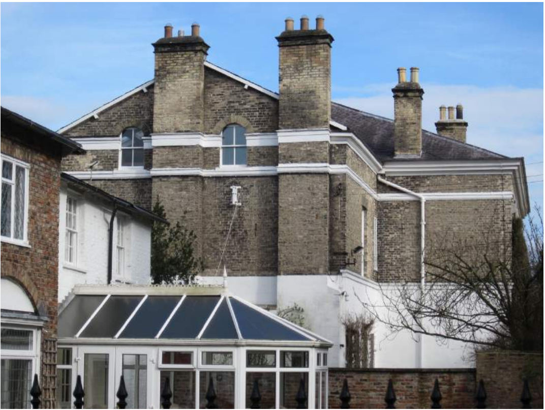
Fig 17 West elevation with evidence of demolished single-storey service range
