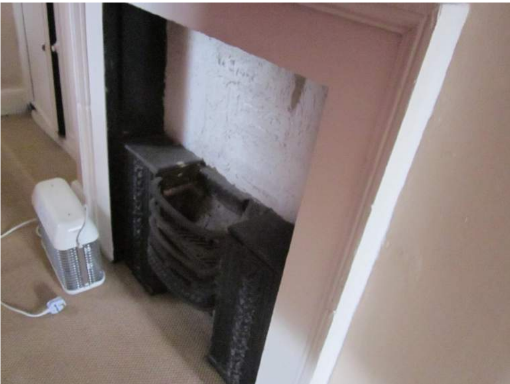
Fig 7: Bedroom 4: Phase I fireplace in contemporary surround
