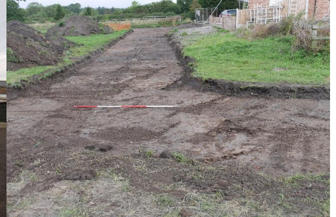
Figure 26: Access Road after stripping looking north-west.
