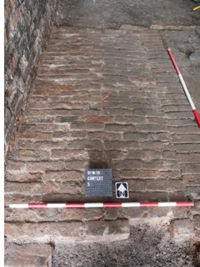
Figure 11: Original Brick Flooring Context (5), sealed under C20th century concrete surface, Context (1) and made-up ground Context (2).
