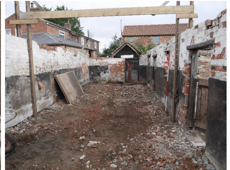
Figure 17: Internal aspect of the Cow House after the removal of the roof and concrete flooring.
