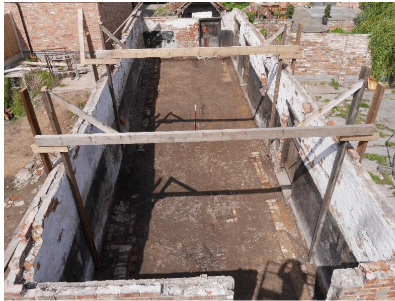
Figure 19: Internal view of Cow House looking north.
