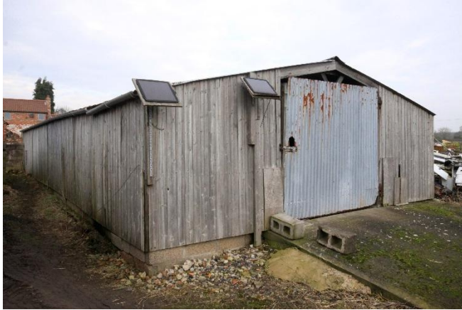
Figure 24: Storage Building 1 looking north-east.
