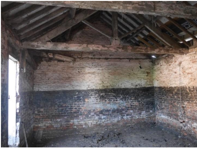
Figure 12: Details of the King Post Roof Construction Typical of All Three Buildings.
