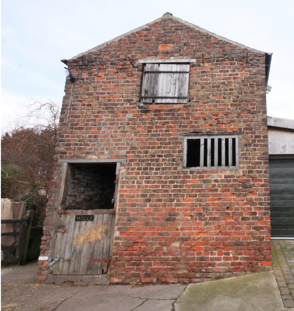
Figure 9: South Facing Elevation of the Combination Barn.
