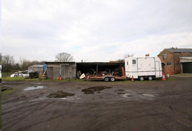
Figure 25: Storage Building 2 looking west.
