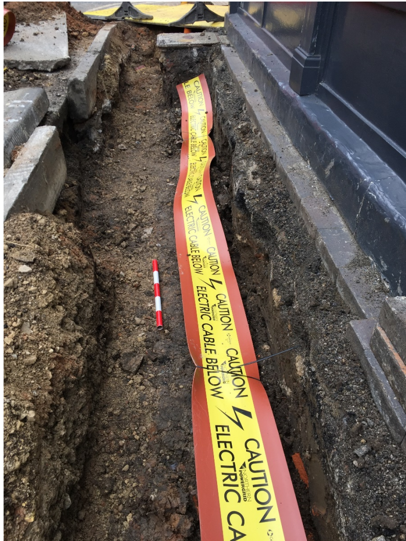
Plate 3 Excavated trench, looking north, 0.1m scale units
