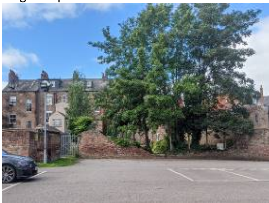
Rear of 26-32 Clifton, St Peter's Terrace
