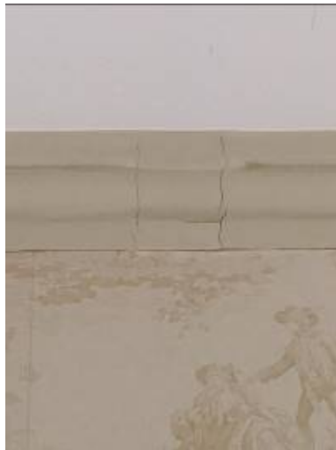
R10 Partition infill in the cornice
